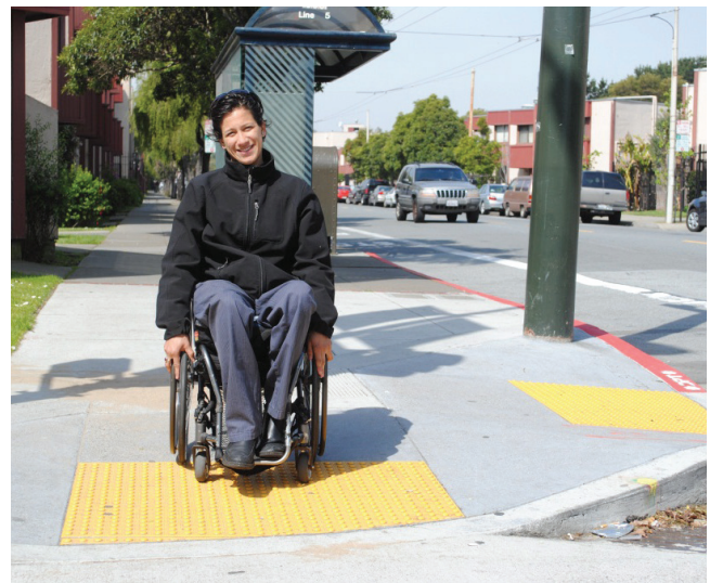
ADA curb ramp with truncated domes
