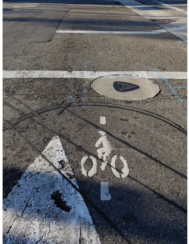
Bicycle detector pavement marking
