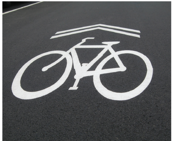
Shared lane “sharrow” marking
