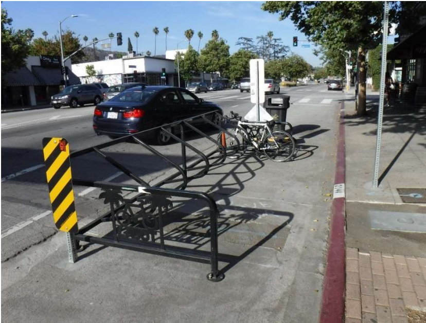
Figure 28. This bicycle corral utilizes the area of a single parking space to provide parking for up to six bicycles.
