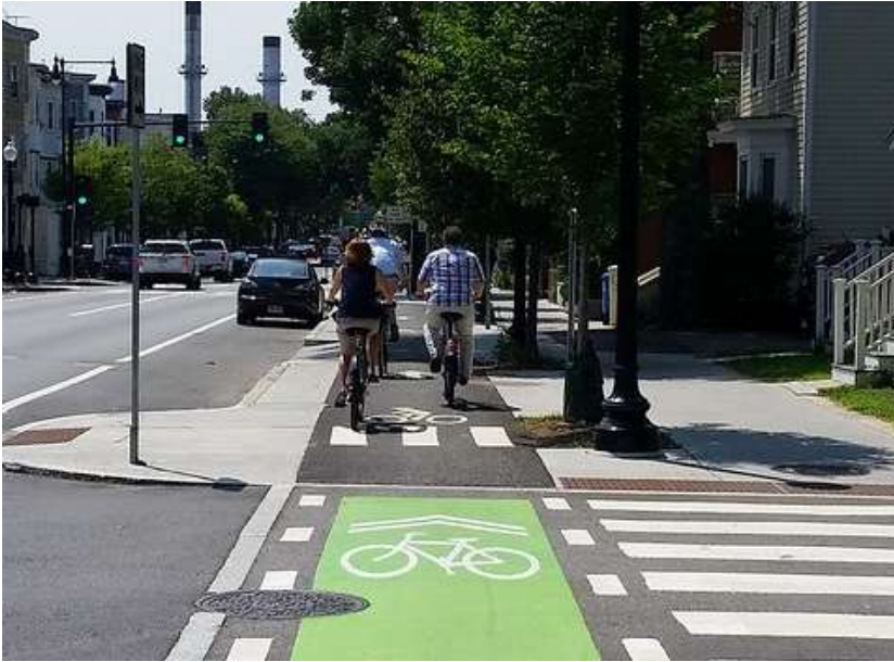
Figure 27. This separated bikeway example in Cambridge, Massachusetts is separated from the vehicle lanes by on-street parking and loading area, and from the parallel sidewalk by a row of shade trees.
