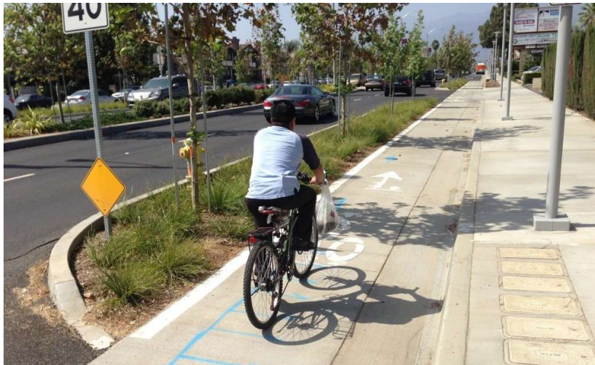
Figure 34. In this example, bioswales buffer the bike lane from the vehicle lanes, creating a Class IV separated bikeway.
