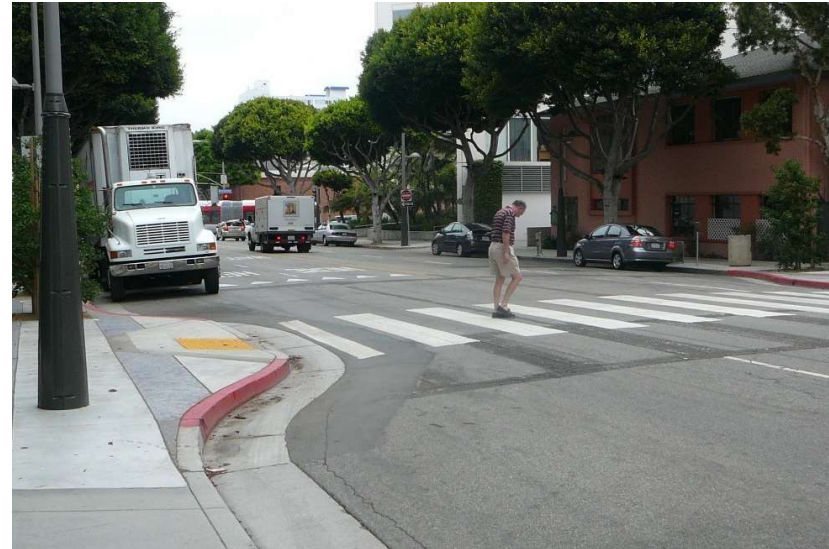
Figure 30. These curb extensions on either side of the street shorten the crossing distance.
