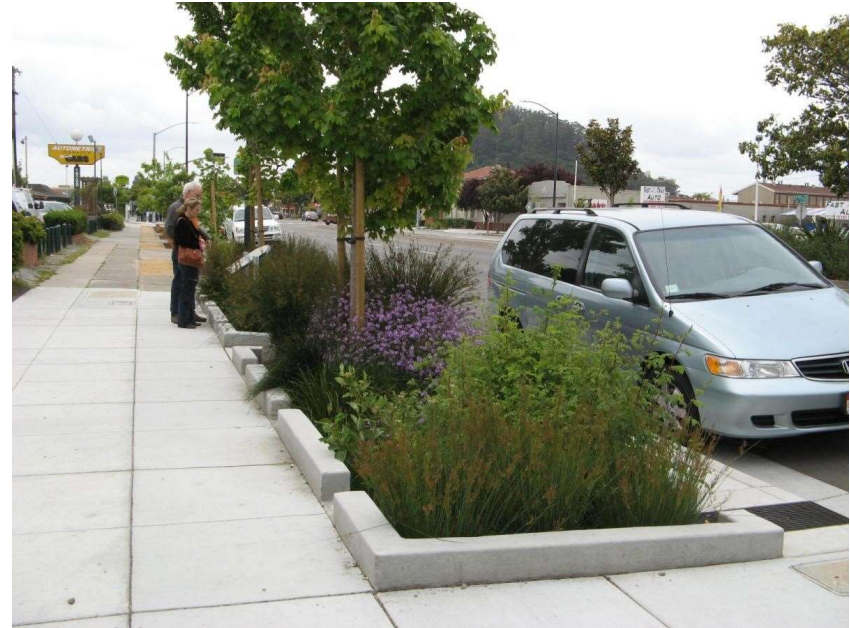
Figure 35. This rain garden buffers the sidewalk from adjacent travel lanes, adds shade to the pedestrian realm, and help recharge groundwater supply by funneling stormwater directly into the ground.
