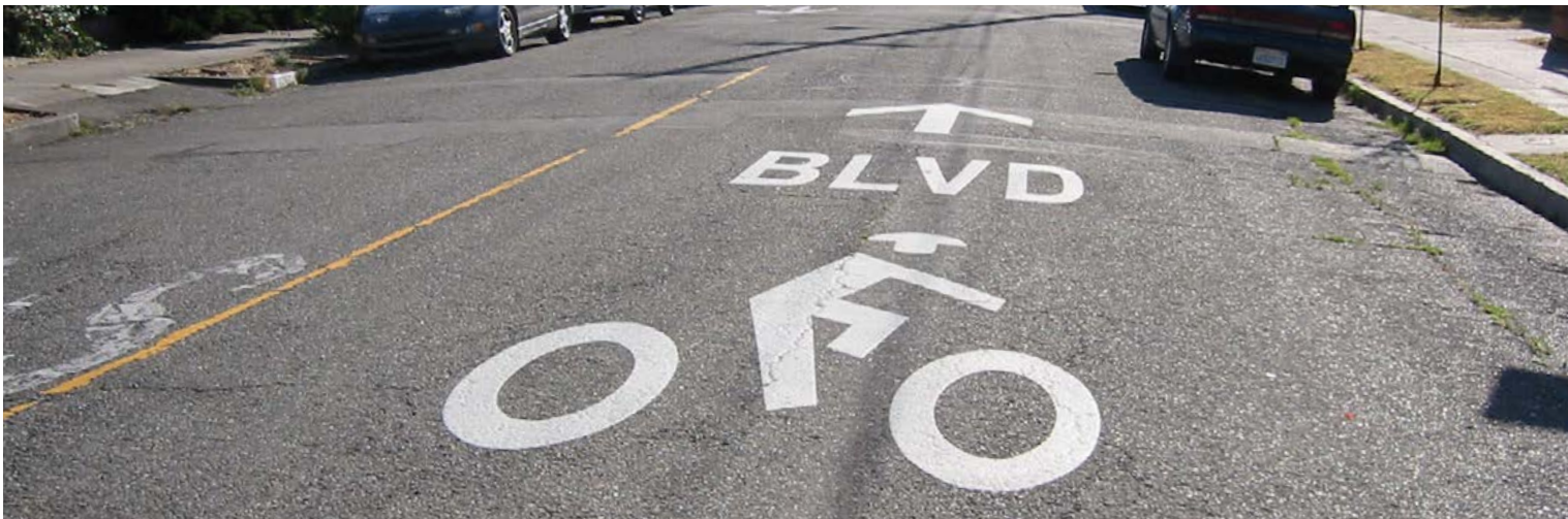
Wide “bicycle boulevard” stencil in Berkeley, CA, takes up most of the lane width. Source: NACTO
