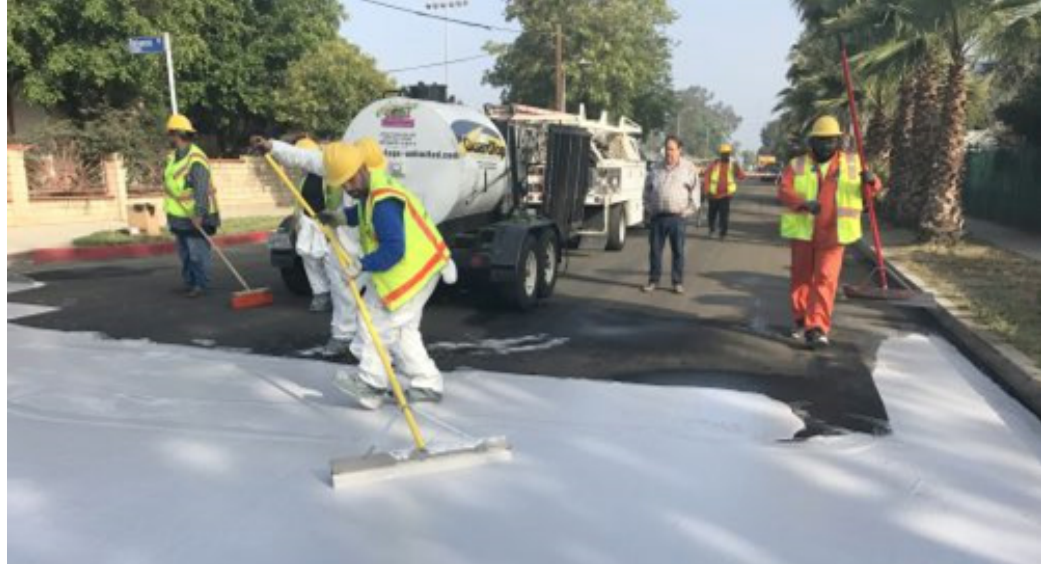
Public works employees apply a cool paving treatment in Los Angeles.
