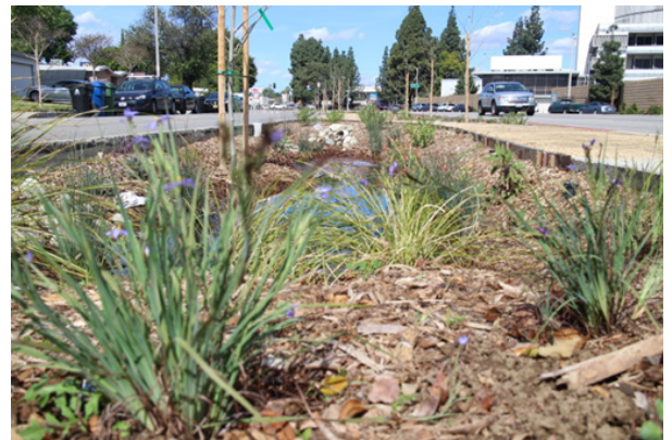
Stormwater Bio-Swale. Source: scpr.org
