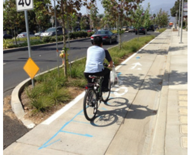
Durfee Avenue in South El Monte, CA, a community in the San Gabriel Valley whose climate is similar to Arvin. Here curb extensions capture and clean water and provide shade.
