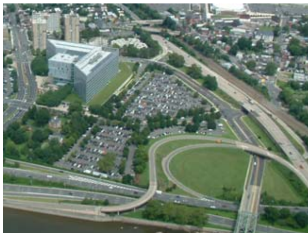
Fig. 17: Intersection on Route 29, Trenton NJ – Before.
