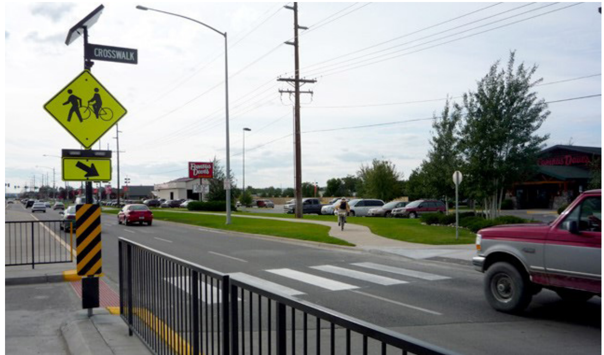
Example uncontrolled bicycle and pedestrian crossing with RRFBs
