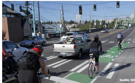
Green Conflict Zone Striping
