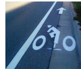
Bicycle lane painted over gutter pan
