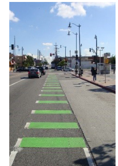
Green skip-striping at intersection where cars may merge across or into the bicycle lane
