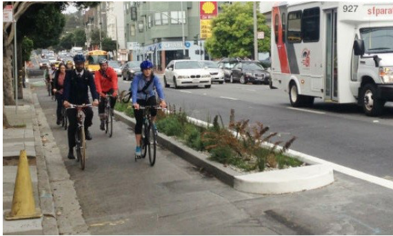
Bikeway separated by landscaping and raised concrete curb
