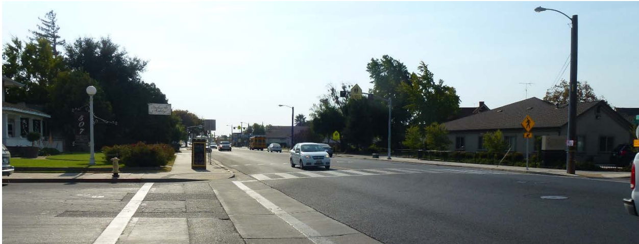
Crosswalk markings are inconsistent, with some continental markings and some transverse
