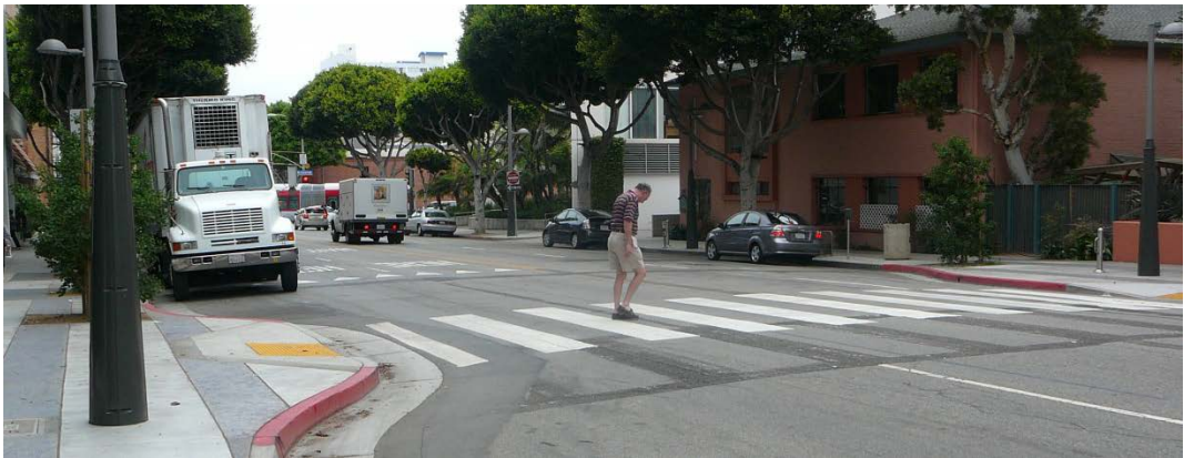
Curb extension with high visibility crosswalk
