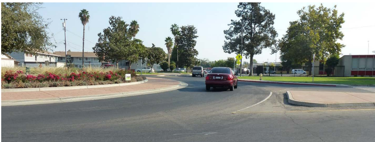
Wide lanes and insufficient horizontal deflection allow high speeds at a roundabout
