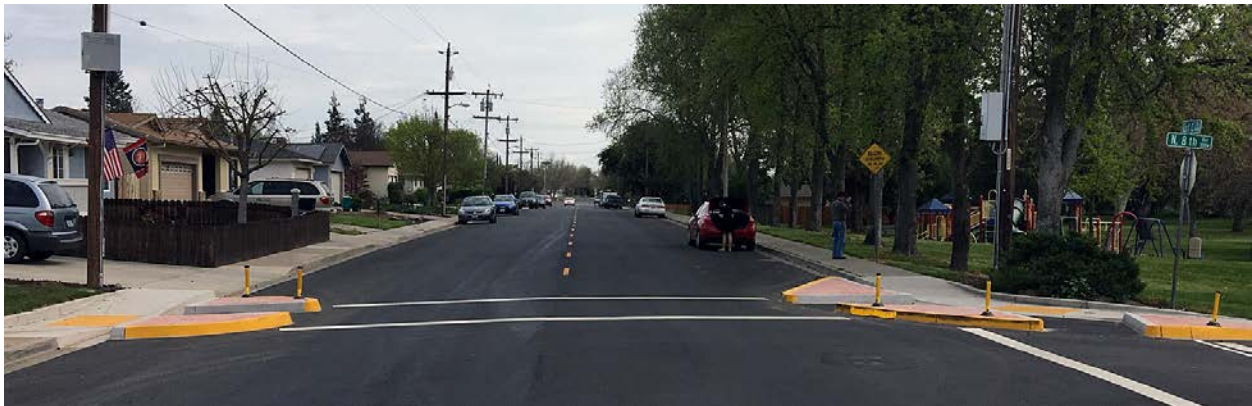
The City of Oakdale installed curb extensions at the intersection of E C Street and N 8 th Street to reduce crossing distances for pedestrians and reduce the turn radius for people driving
