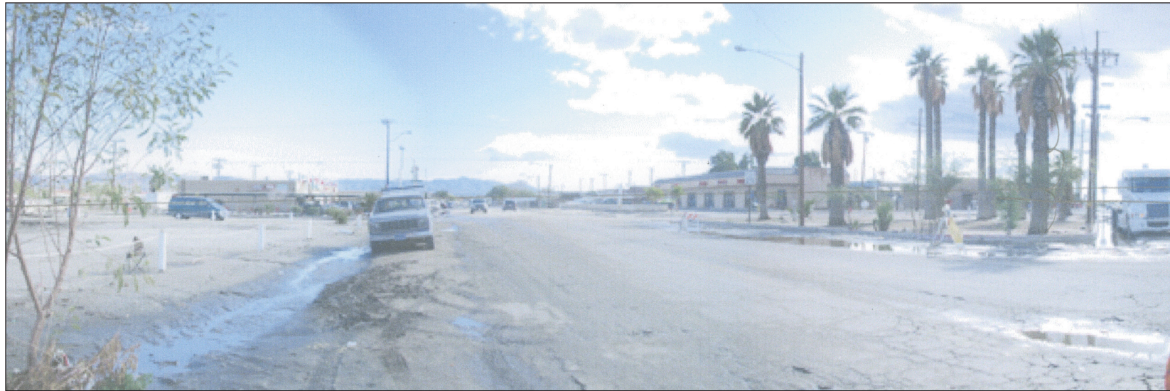
Above: View of existing 2nd Street (at Hammond) looking east
