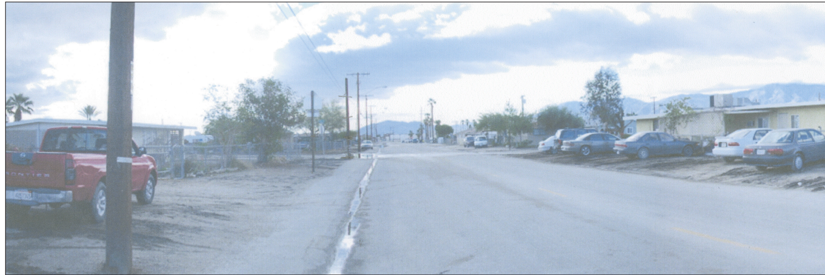
Above: View of existing Coahuilla Street looking South
