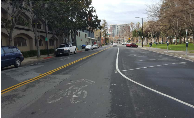
Figure 6-14: Diagonal parking with buffer space and shared-lane marking in San Jose, CA (not a state highway)
