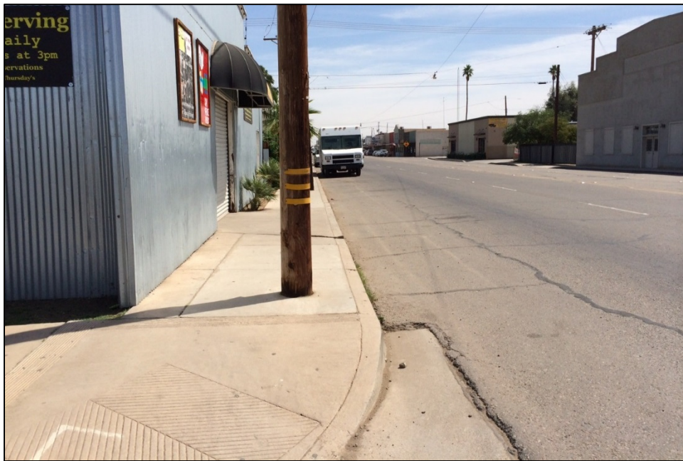
Figure 4-14: Northeast corner of Cedar Avenue and Fifth Street, looking east
