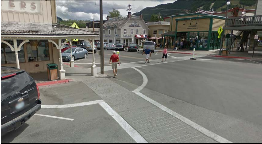
Figure 6-17: Interim curb extensions in Jackson Hole, Wyoming
