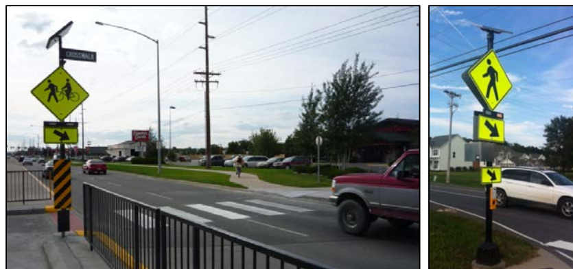
Figure 6-26: RRFB in median crossing (left) and at sidewalk edge (right)
