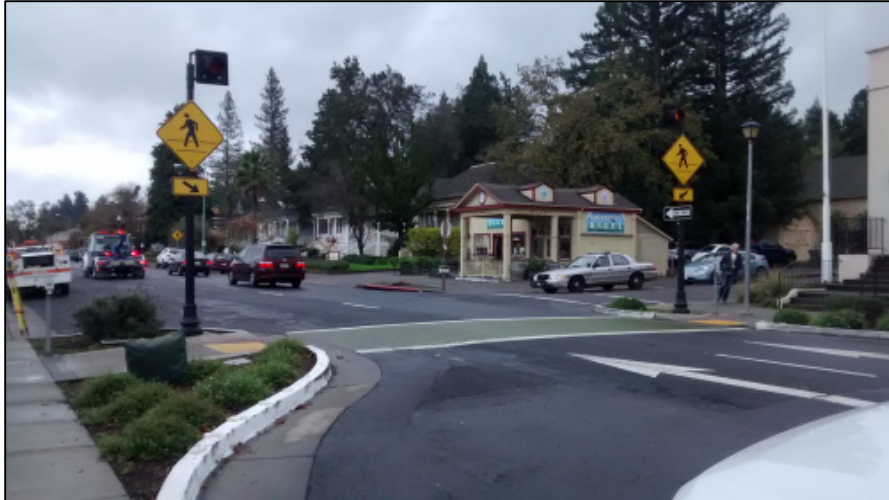
Figure 6-47: High visibility crosswalk on SR 116 in Sebastopol
