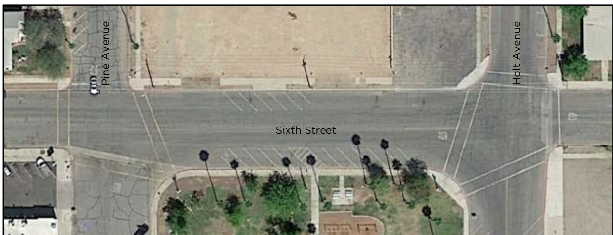
Figure 4-9: Aerial view of Sixth Street at Holt Park
