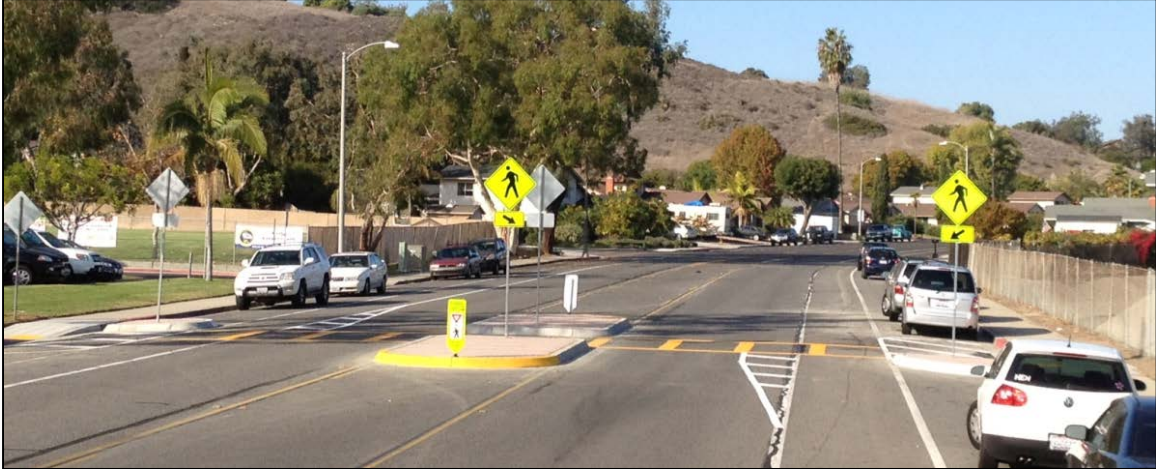
Figure 6-11: Pin-down concrete medians are a lower-cost and quicker solution
