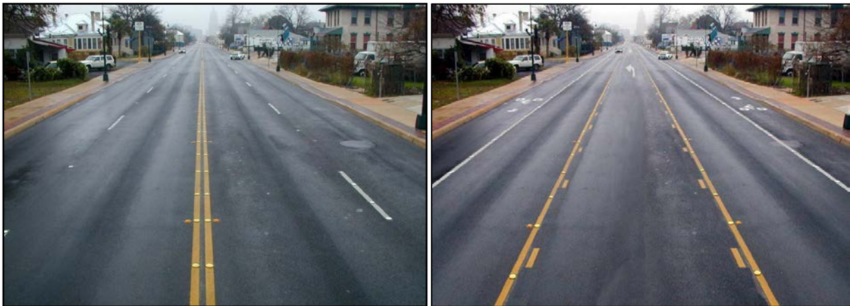
Figure 6-9: On the left: a four lane roadway. On the right, a five lane roadway: three vehicle lanes and two bicycle lanes
