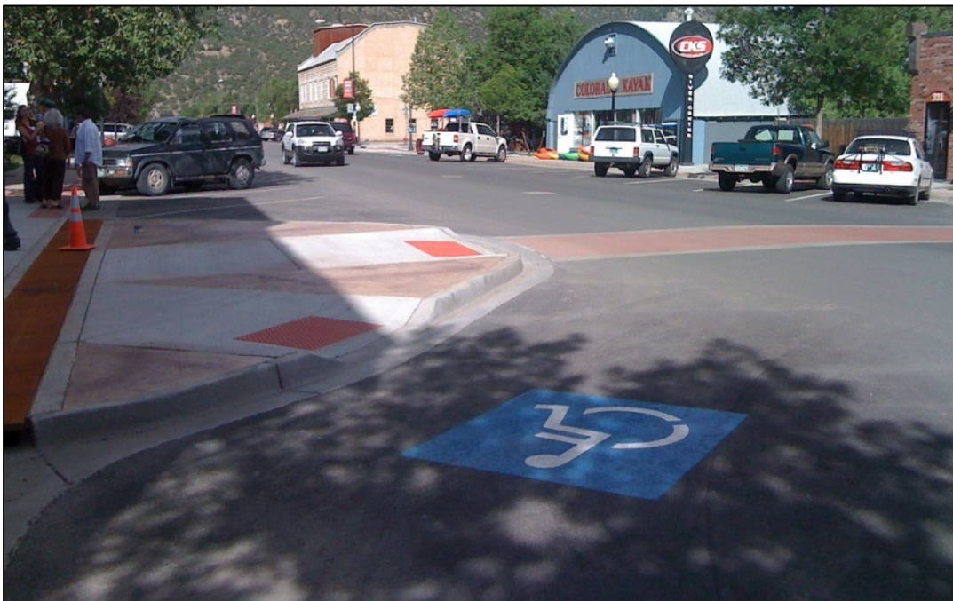
Figure 6-16: Curb extensions in Colorado
