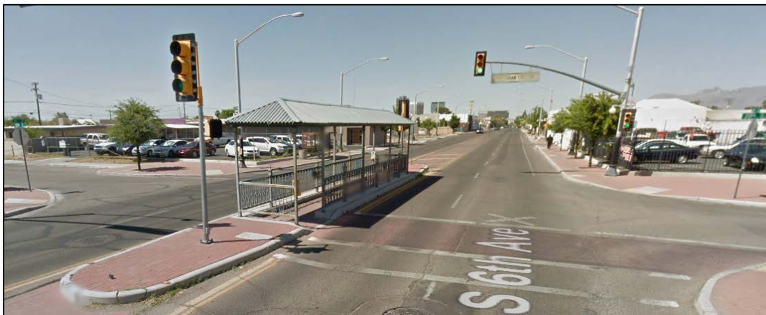
Figure 6-50: Two-stage Pelican crossing in Tucson, AZ
