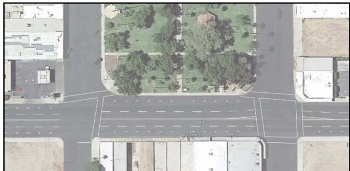
Figure 6-7: Enhanced aerial view of Fifth Street at Holt Park shows a crosswalk leading to another crosswalk, which do not conform to Caltrans standards
