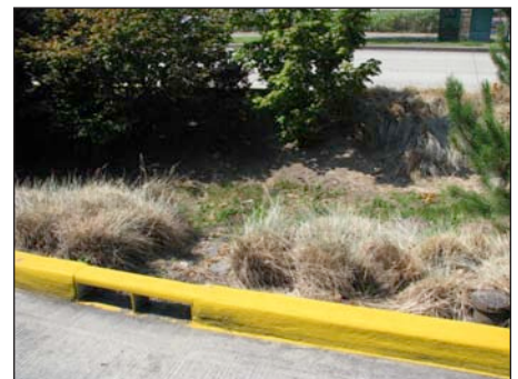
Above (from top to bottom): A landscaped bulb-out with parallel parking; An example of painted bike lanes and center median; An example showing street drainage and a rain garden condition.
