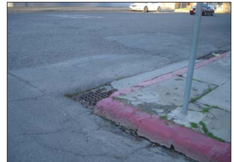
Above (from top to bottom): Existing view of Blossom looking east towards downtown shows an expanse of empty pavement; Existing view of Blossom approaching Center Avenue; Existing infrastructure is in need of maintenance and lacking pedestrian facilities such as curb ramps and crosswalks.
