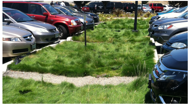
Vegetated swales, such as this installed in a parking lot, can both treat and convey runoff, eliminating the need for some catch basins and pipes.
