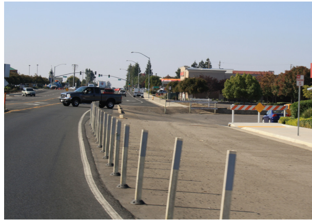
SR108 has many sections with significant unused right-of-way area ideally suited for LID treatment facilities.
