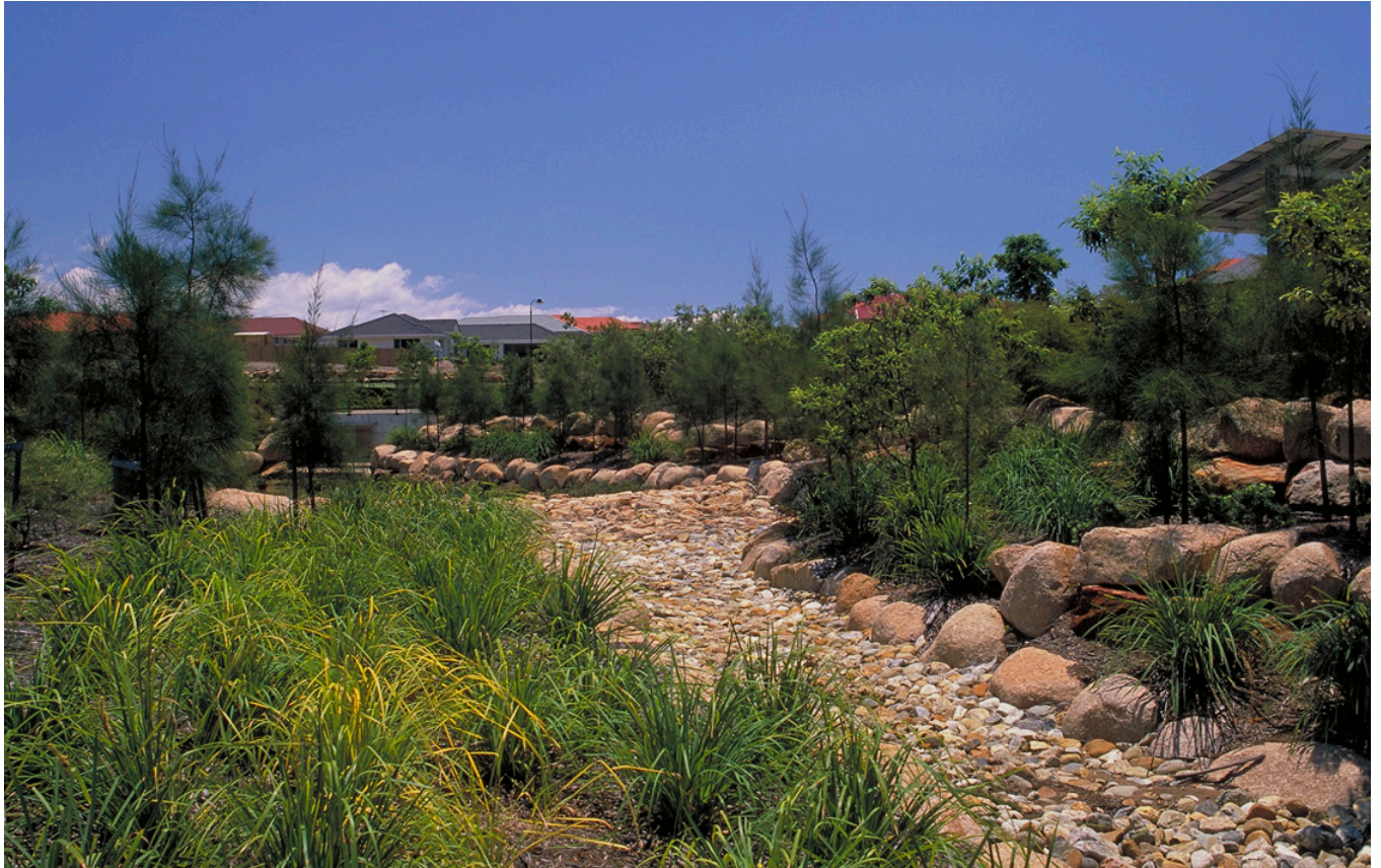
The deployment of BMPs on a site can take many forms, which allows the facilities to integrate with landscaping while still providing optimal stormwater functionality. These examples show bioretention areas within an outdoor courtyard (above left), a vegetated swale and filter strip serving as a buffer for homes (above right), and a rocky swale area meant to be appealing while dry but able to handle infrequent large flows.
