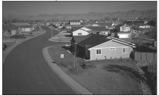
Conventional development near Las Vegas, Nevada.
