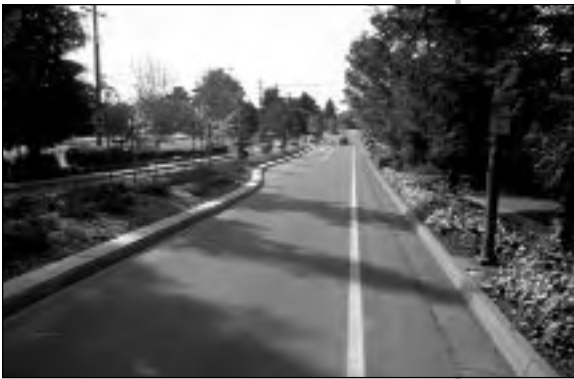
An avenue in Mountain View, California with a median, 12-foot travel lanes, 5-foot bike lanes, planting strip, and sidewalk setback from the roadway. High capacity is handled at each intersection, where
