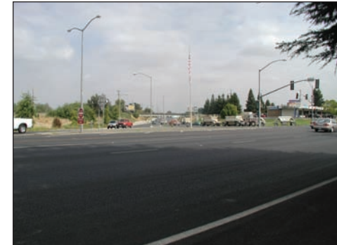
The intersection looking east from North Beale Rd.
