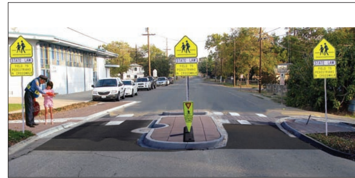
Curb extensions and a pedestrian refuge island are added for safe crossing and ensuring cautious speeds before, during and after school hours.
