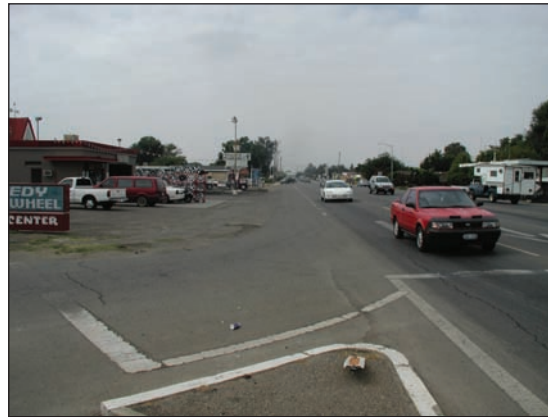
Missing sidewalk, undefined edge and broad corner allows high turning speeds and creates imposing conditions for pedestrians.
