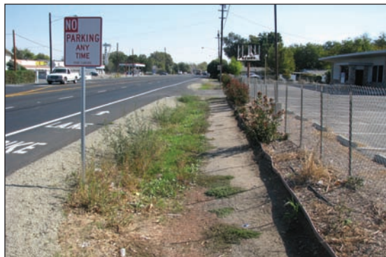
Before: North Beale Road looking east.
