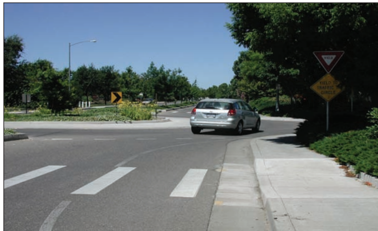
Photo at top shows the basic parts and functions of a roundabout. Bottom shows how deflection causes driver to slow down.
