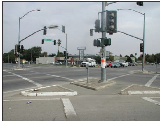
Driveway location, crosswalk placement and the design of right-hand slip lanes at the intersection of North Beale and Hammonton-Samrtville roads produce many conflicts and hazards for motorists, pedestrians and bicyclists.
