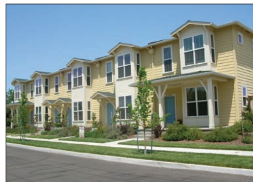
Townhomes next to four-lane road in Chico, California.
