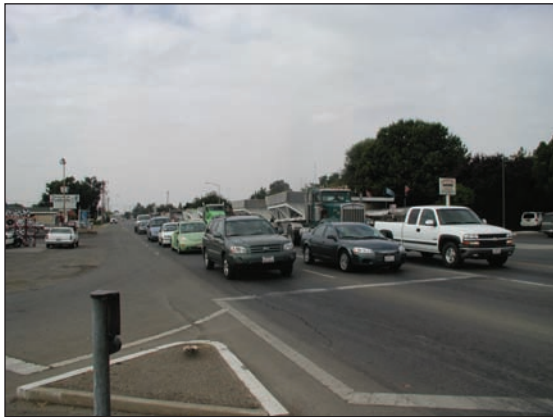
Missing sidewalk, undefined edge and broad corner allows high turning speeds and creates imposing conditions for pedestrians.
