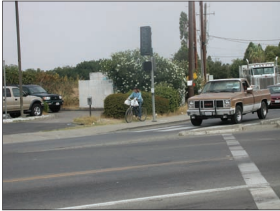
Driveway location, crosswalk placement and the design of right-hand slip lanes at the intersection of North Beale and Hammonton-Samrtville roads produce many conflicts and hazards for motorists, pedestrians and bicyclists.
