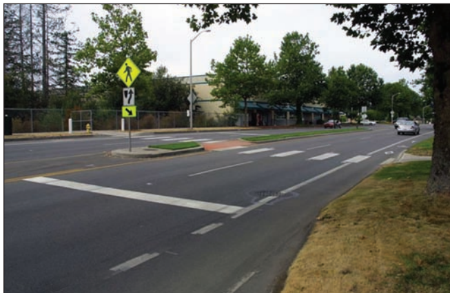
Refuge island with high visibility crosswalk (longitudinal striping) and stop bar. Sign placement and high contrast materials helps ensure motorists will see the center island.
