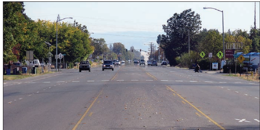
The wide roadway, high traffic speeds and absence of sidewalks creates a stark and imposing environment for pedestrians and motorists.
