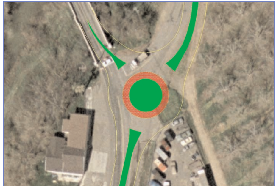
Concepts for roundabouts on north (top) and south (bottom) ends of the Putah Creek Bridge.
