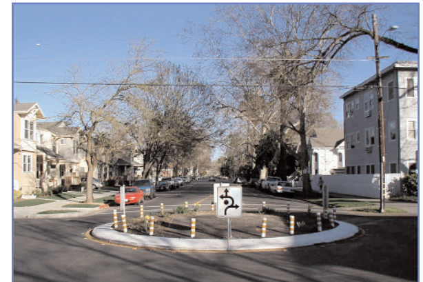
Mini-circles are used to slow traffic on both approach streets. Although not shown in this photo, crosswalks should be marked and curb ramps provided on all four corners.
