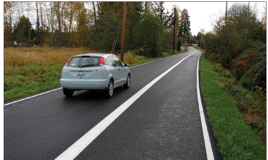
A “Scenic Slow Road” in Lake Stevens, Washington limits the travel way for cars to one-lane while accommodating non-motorized users in a separate lane.
