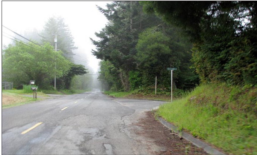
The absence of shoulders makes for unsafe conditions for non-motorists
