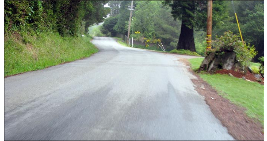
Westhaven Drive without Centerline
