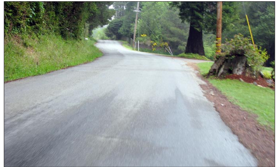
Westhaven Drive without centerline
