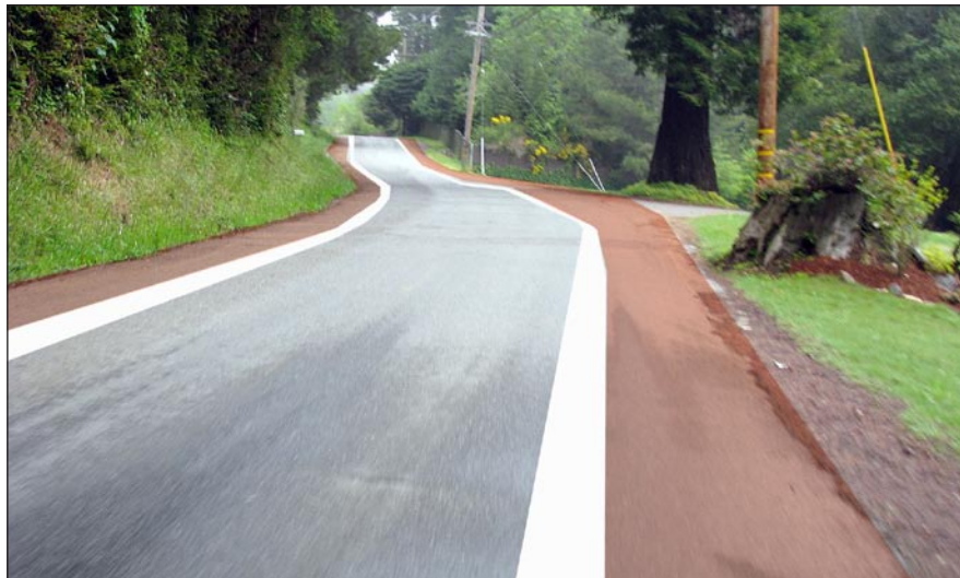
Colorized shoulder and narrow travel way are signatures of Scenic Slow Road options
