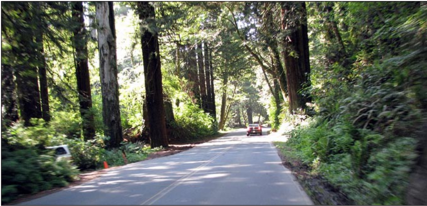
Some areas along Scenic Drive are stable and allow two-way travel lanes
