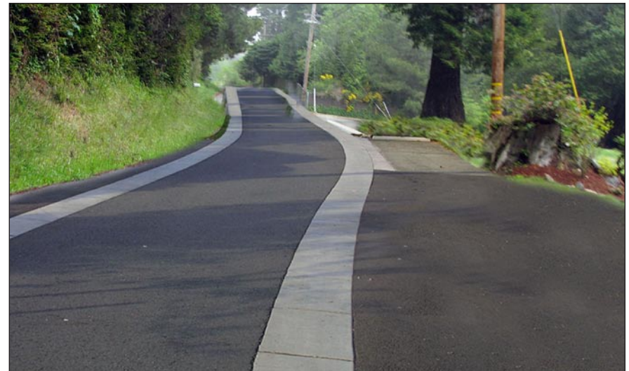
Where the travel way is limited to one way, a pullout allows for safe passage at slower speeds
