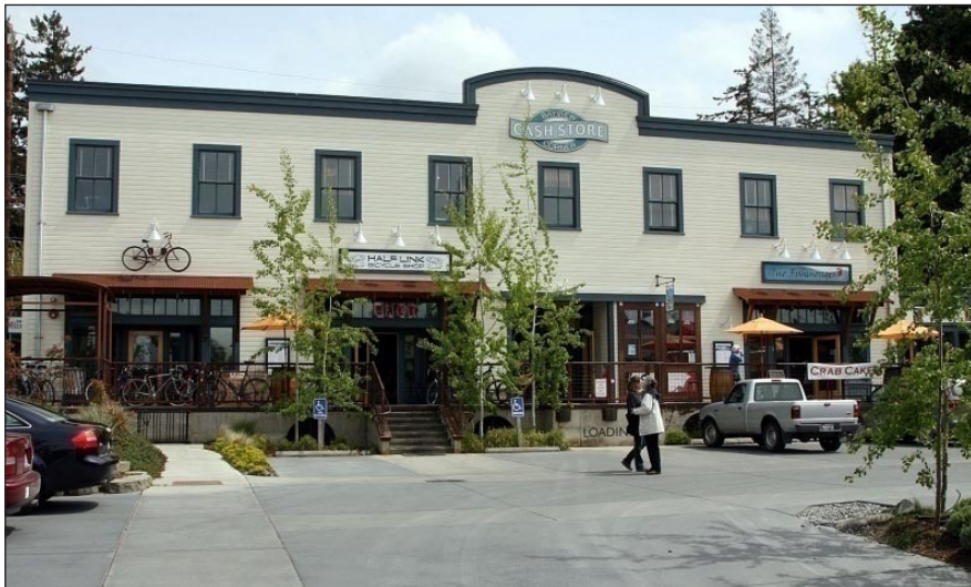
A convenience store (mini-mart) with office or housing space on the second floor is another “Smart Growth” option
