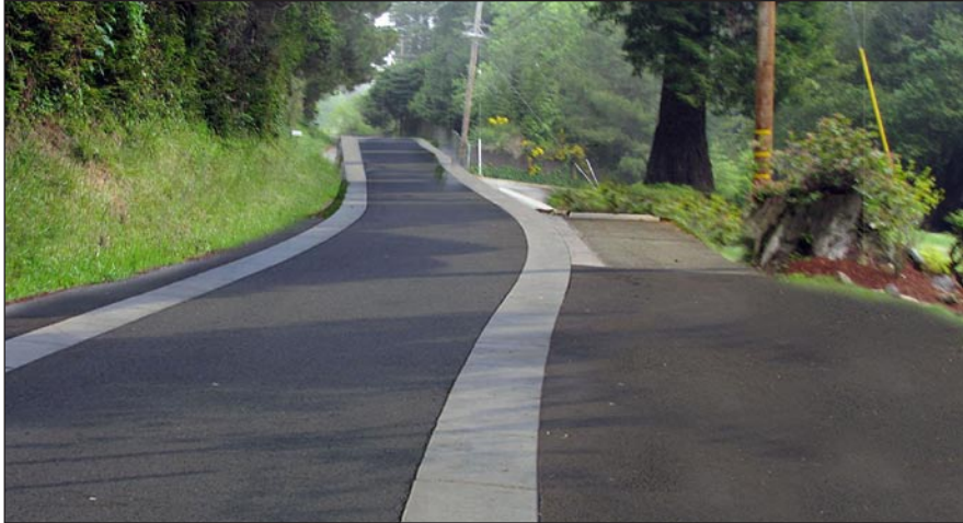
Where the travel way is limited to one way, a pullout allows for safe passage at slower speeds
