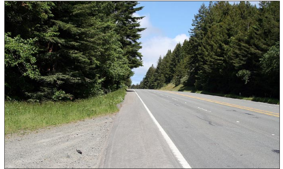
Northbound Highway 101 approaching crest of hill
