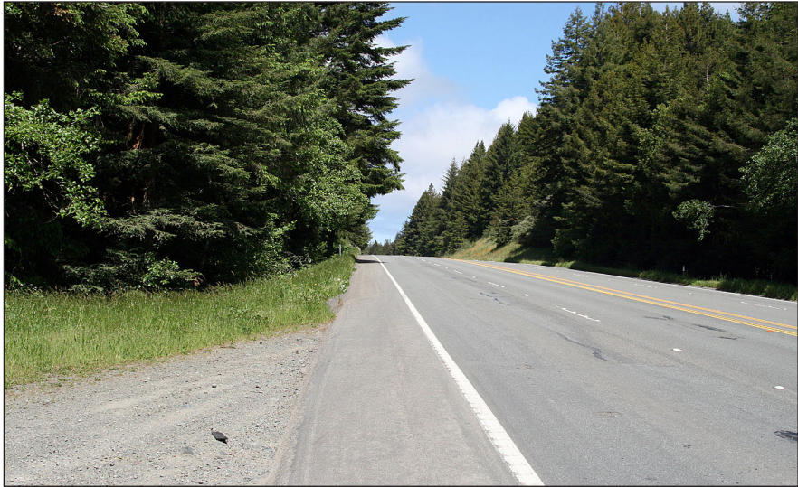
Northbound Highway 101 approaching crest of hill
