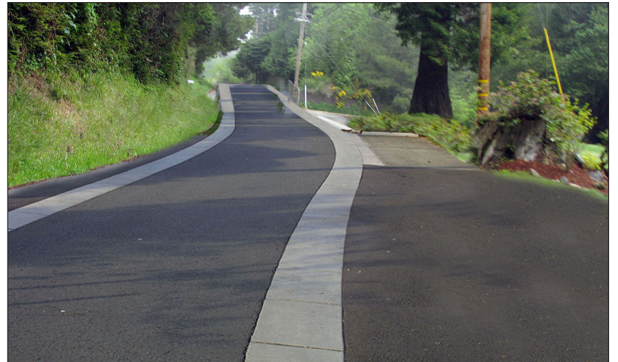
Where the travel way is limited to one way, a pullout allows for safe passage at slower speeds
