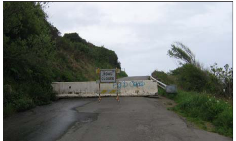
Road closure after 2006 winter storm
