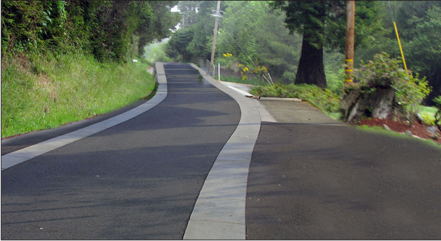
Where the travel way is limited to one way, a pullout allows for safe passage at slower speeds
