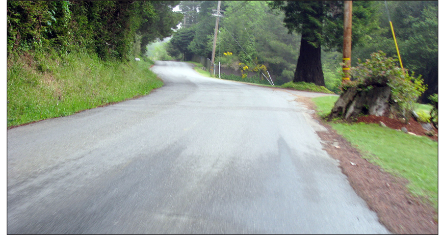
Westhaven Drive without Centerline
