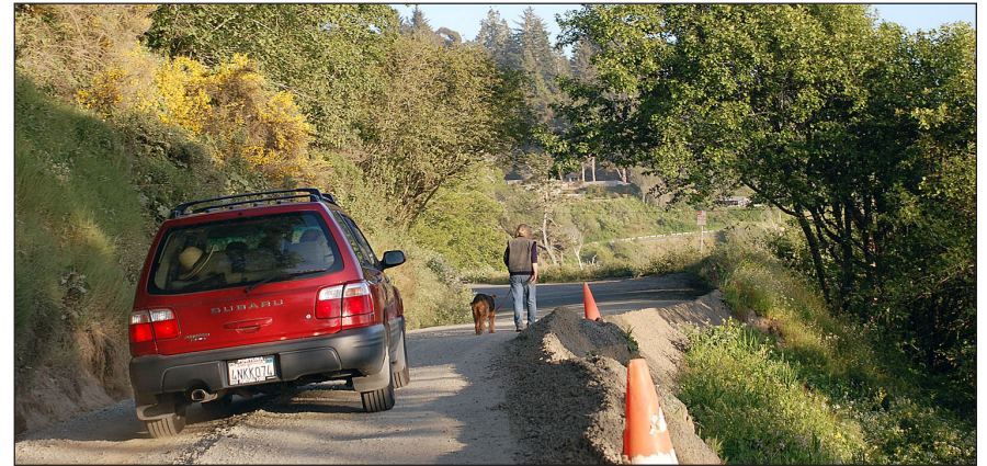
In many cases, slope failures require a much slower speed to allow cars and pedestrians to co-exist safely
