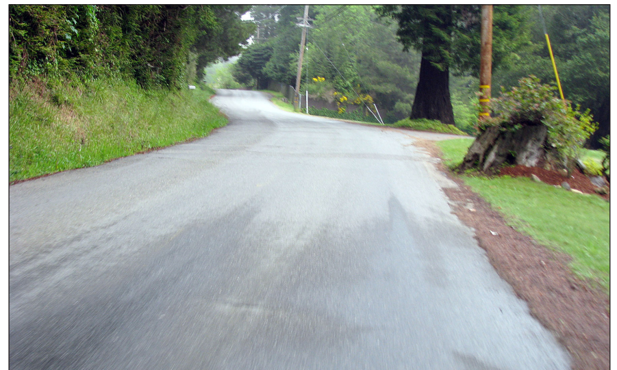
Westhaven Drive without centerline
