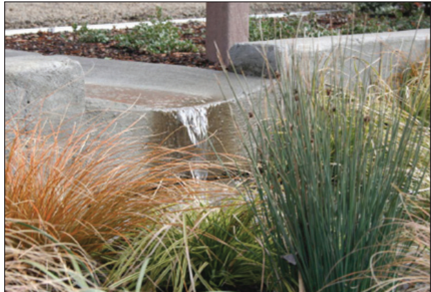
Above Left: Currently, storm water drains to drop inlets which are connected to pipes that convey the water downstream. Above Right: Stormwater drains to a bioretention facility which slows runoff and provides initial filtering.
