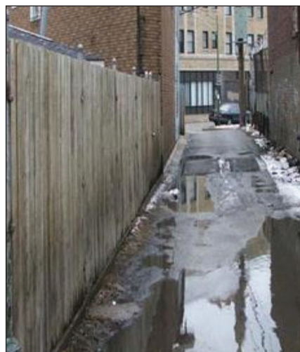
Bottom Left to Right: Impervious surfaces cause stormwater to “pond” before running off. Permeable surfaces allow stormwater to infiltrate into the ground below.
