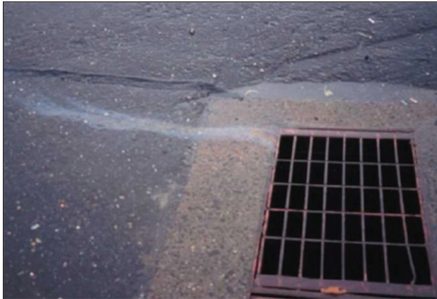
Above Left: Currently, storm water drains to drop inlets which are connected to pipes that convey the water downstream. Above Right: Stormwater drains to a bioretention facility which slows runoff and provides initial filtering.
