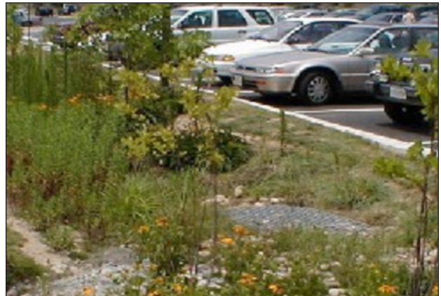
Above Left: At a larger scale, runoff can be directed to drainage swales that retain and provide initial treatment.
