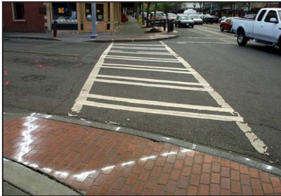
ADA requirements were often originally met in haste without proper alignment of paths. Many municipalities are now correcting these placements.
