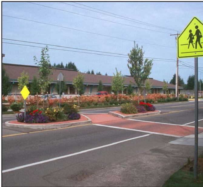
An example of a good mid-block crossing.
