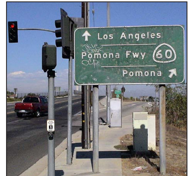
Pedestrians face multiple obstacles on sidewalks.
