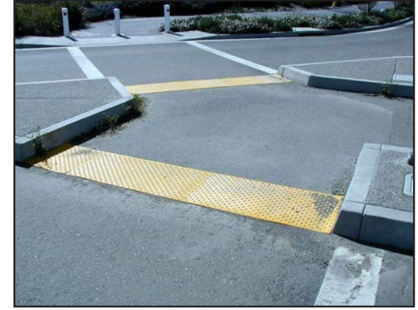
Tactile edges allow the vision-impaired to sense the edge of the “safe zone” for pedestrians and know they are crossing traffic.
