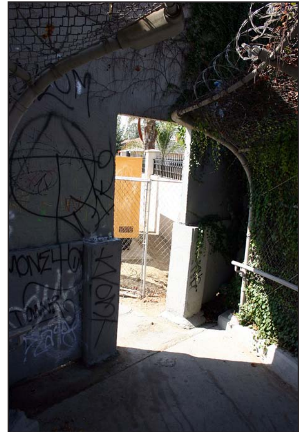
Unsafe and unsightly — not South El Monte's standard.
