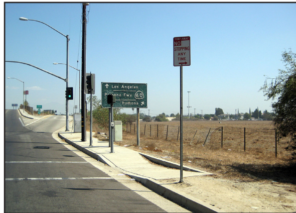
Once at Hwy 60, we see ADA ramps, but many poles.
