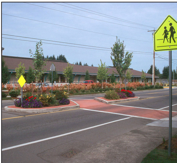
An example of a good mid-block crossing.
