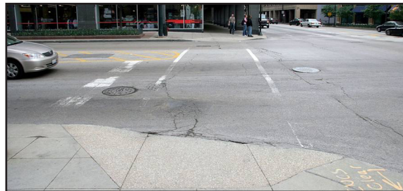
Crossing enhancements (especially stripes) should be maintained to draw motorist attention to pedestrian zones. Crossings that are not maintained lead to less certain (and less visible) pedestrian paths.
