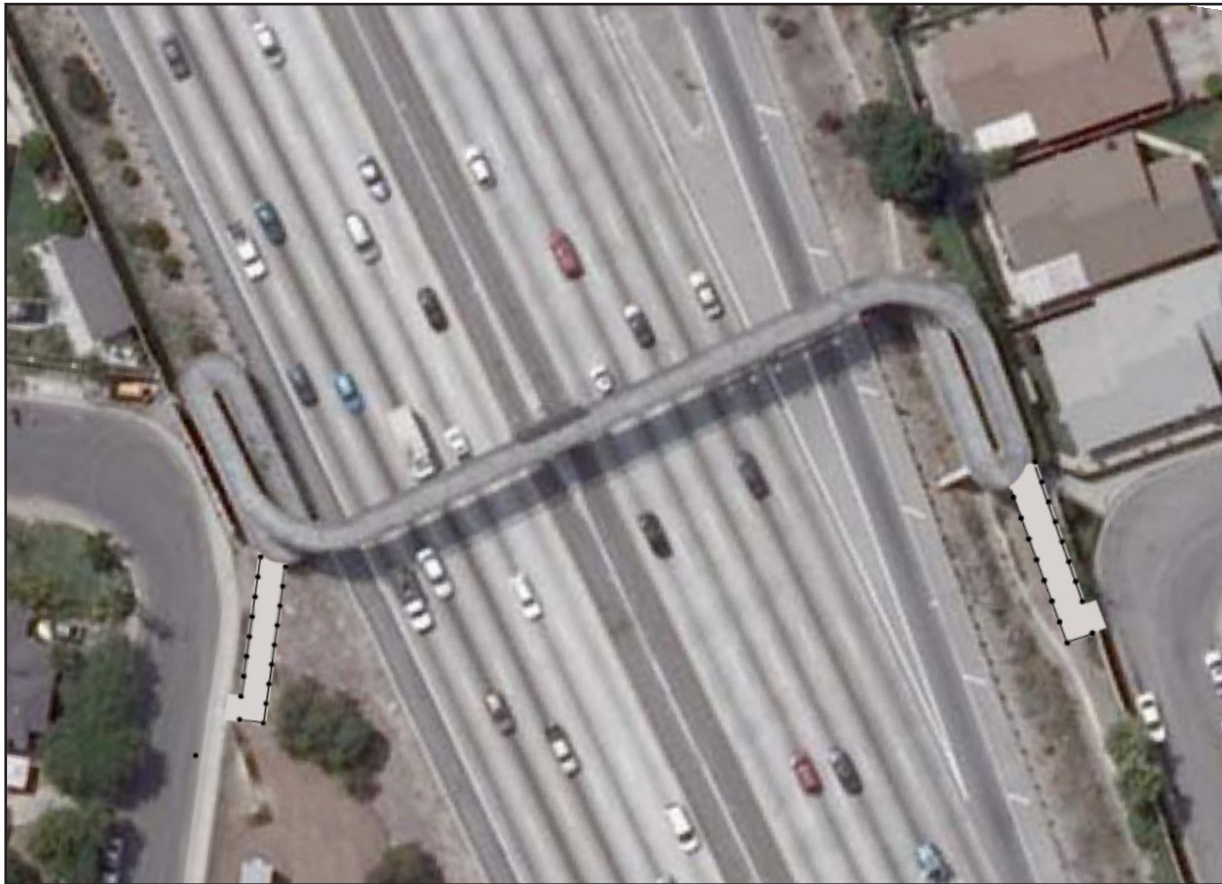
Figure 3-23: New entryway ramps at both ends of the high school overpass structure.
