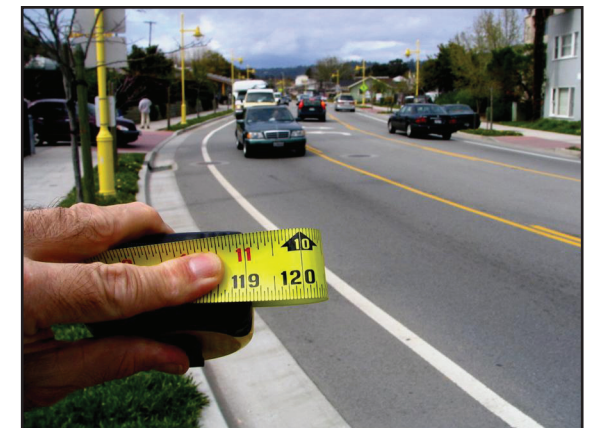
10-foot travel lanes provide a good balance between vehicle and pedestrian safety and comfort.
