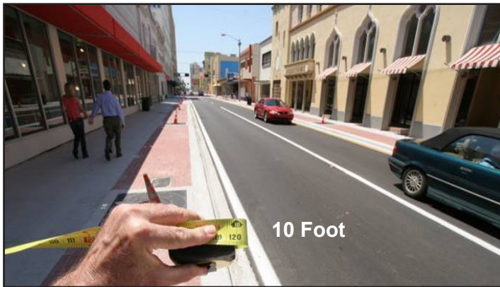
Olive Avenue. Lanes were narrowed to 10 feet in downtown West Palm Beach, Florida in 2005-06. This city is now completing a series of lane width reductions on four different typical sections of Olive Avenue (formerly 3 to 5 lanes wide).
