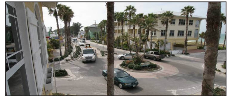
Installation of a roundabout calmed traffic speeds and facilitated pedestrian crossing. It also improved property values and catalyzed redevelopment.
