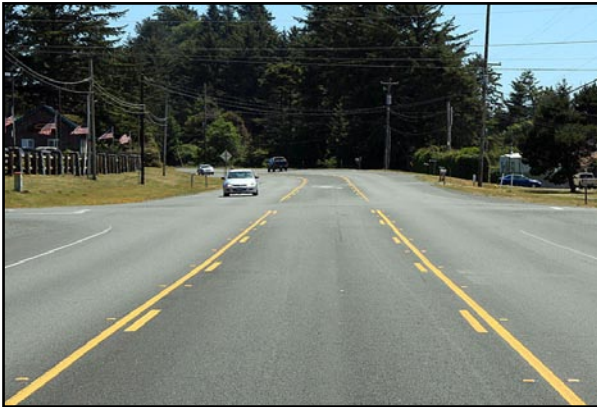
For northbound traffic, a pronounced curve limits the view of the upcoming intersection of Highway 101 and North Indian Road.
