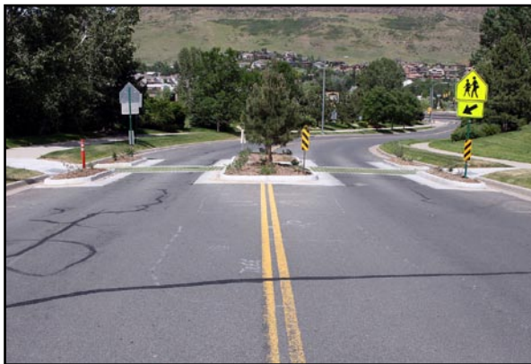
Raised curbs and landscaping extend the narrowing effect of striping and colorizing by adding a vertical dimension.
