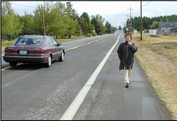
Widening all shoulders to a minimum of 8 feet would provide more room for pedestrians and bicyclists.
