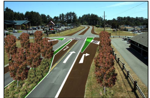
Dedicated turn lanes allow the motorist to make safe turns in a timely manner.
