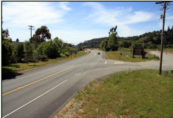
Curves in the alignment of Highway 101 limit distant views of Rowdy Creek Road for both north and southbound traffic.
