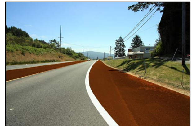
Colorizing the shoulder can further delineate a change in roadway conditions that will require a corresponding change in motorist behavior.
