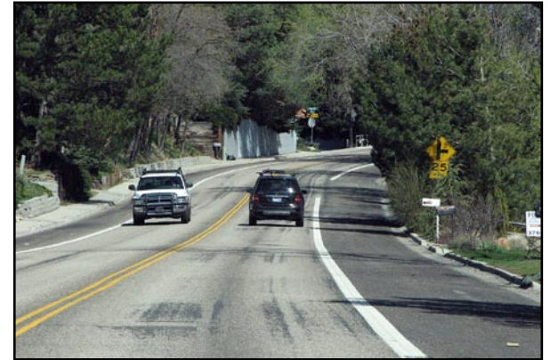
Widening the fog line or bicycle lane line from the typical 4-inch wide stripe to an 8-inch wide line alerts the motorist that the roadway is changing.
