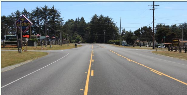
Existing intersection at North Indian Road and Highway 101.
