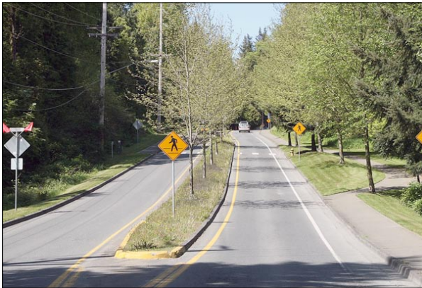
Landscaping can also be used to indicate to motorists that they are entering a new environment and should slow down.
