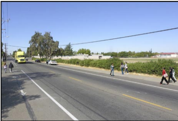
Widened shoulders on Hurley Way in Sacramento, County, CA. Steve Price Urban Advantage.
