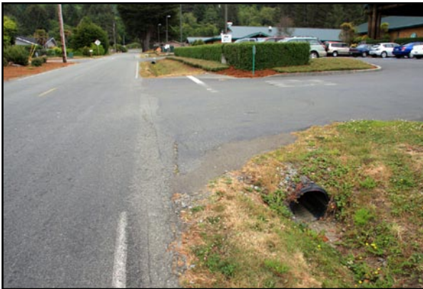
Sidewalks should be installed on both sides of North Indian Road from Oceanview Drive to Highway 101.
