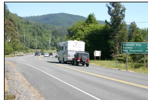
Highway 101 is the principal highway in the region.
