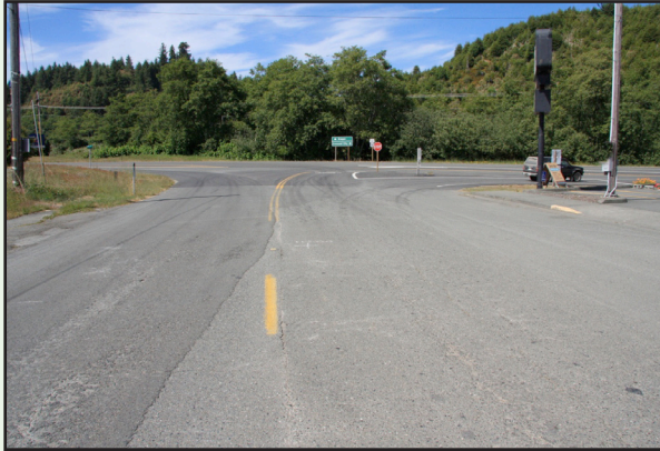
Existing intersection at Fred Haight Drive and Highway 101.
