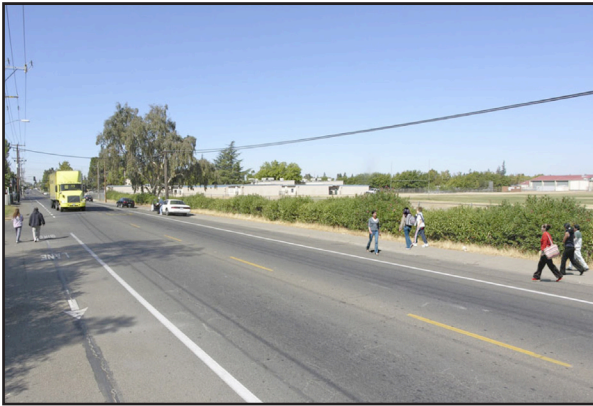
Widened shoulders on Hurley Way in Sacramento, County, CA. Steve Price Urban Advantage.
