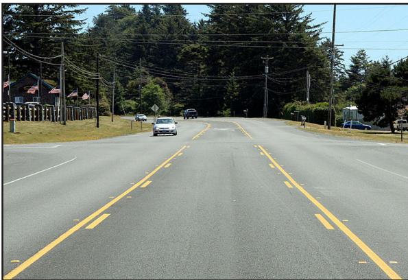
For northbound traffic, a pronounced curve limits the view of the upcoming intersection of Highway 101 and North Indian Road.
