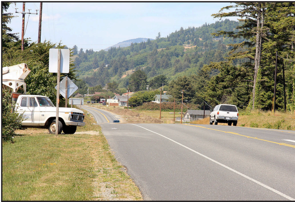
For southbound traffic, a hill restricts the view of the upcoming intersection of Highway 101 and North Indian Road.
