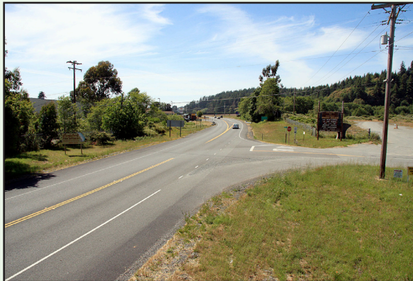
Curves in the alignment of Highway 101 limit distant views of Rowdy Creek Road for both north and southbound traffic.
