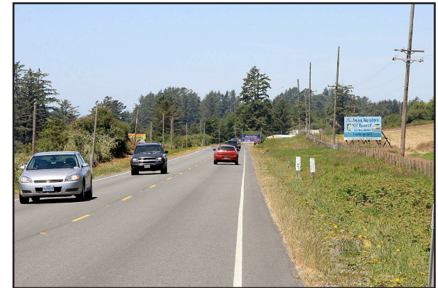
Inadequate shoulder widths pose hazards to disabled vehicles, bicyclists, and pedestrians.
