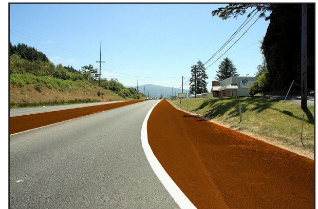
Colorizing the shoulder can further delineate a change in roadway conditions that will require a corresponding change in motorist behavior.
