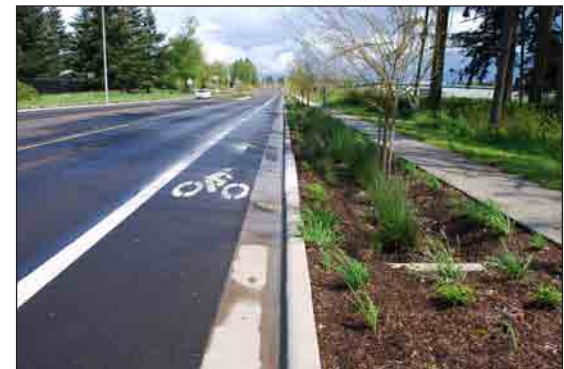
Top left: many bicyclists use the shoulder on Route 1 for commuting, exercise and recreation. Top right: riders choose the shoulder against traffic over the adjacent multipurpose trail. Above: clearly designated lanes and a consistent edge condition like the example above placed on both sides of Highway 1 would provide clarity for motorists and bicyclists alike.
