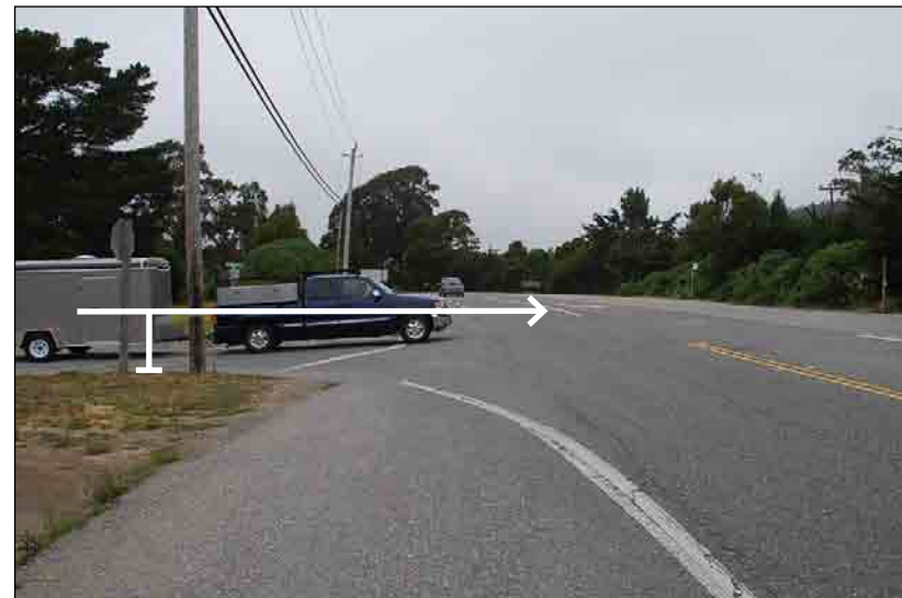
The change in approach grade reduces driver sight distance.
