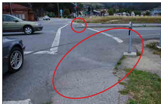
Corner needs to be finished with curb and sidewalk, and median tip should be removed at Capistrano intersection.
