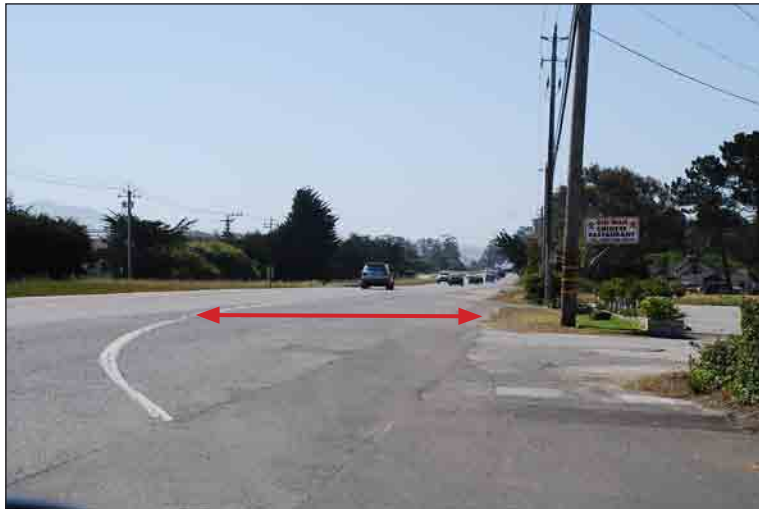
Top: Miramar looking north toward El Granada. Bottom: Miramar looking south. The photos show a lack of consistent built cross section width and characteristics and lack of defined inside and outside edges.
