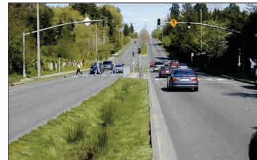
Top Left: Shoulder with stamped, colorized pavement clearly defines road edge on State Highway 16, Capay Valley, Ca. Top Right: landscaped swale delineates the road edge and provides area for natural drainage, and separation between the road and sidewalk. Above Right: raised median with high contrast decorative landscaping. Right: center median designed with a landscaped swale for natural drainage and pedestrian refuge area at a signalized, stop-controlled pedestrian crossing.
