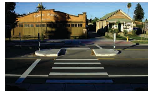
Raised median island with high visibility markings. The stop bar for vehicles is set back from the crosswalk.
