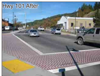
High contrast pavement treatment to highlight the pedestrian crossing area is added to an intersection on Highway 101.
