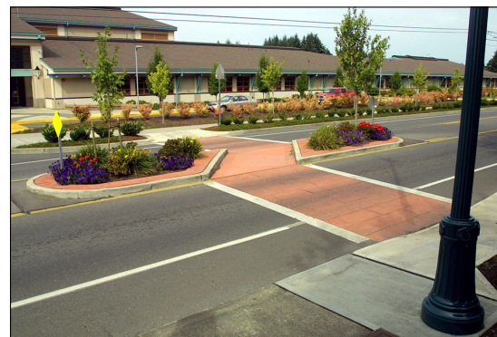
Raised medians allow pedestrians to cross one-half of the roadway and wait in the center for an opportunity to cross the other half. Some raised medians walkways are angled so pedestrians face oncoming traffic before crossing.
