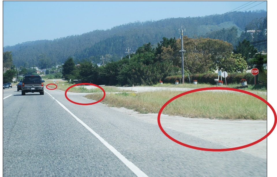
Above: Multiple driveway path openings on Route 1 detract from a consistent edge condition and introduce potential conflicts between turning vehicles and high speed through traffic.
