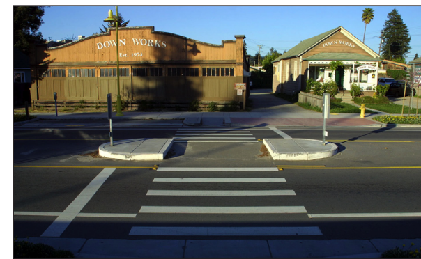
Raised median island with high visibility markings. The stop bar for vehicles is set back from the crosswalk.
