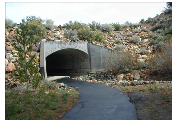
Improvements to the culvert in the top photo could provide a convenient crossing under the highway. If a crossing is developed, it should also accommodate equestrians, although they may need to dismount to minimize height requirements.
