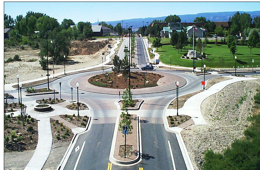
Roundabout size is dependent upon the volume and type of traffic that will pass through the intersection. Roundabouts can be designed to accommodate large trucks.
