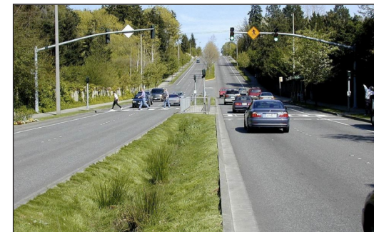
Top Left: Shoulder with stamped, colorized pavement clearly defines road edge on State Highway 16, Capay Valley, Ca. Top Right: landscaped swale delineates the road edge and provides area for natural drainage, and separation between the road and sidewalk. Above Right: raised median with high contrast decorative landscaping. Right: center median designed with a landscaped swale for natural drainage and pedestrian refuge area at a signalized, stop-controlled pedestrian crossing.
