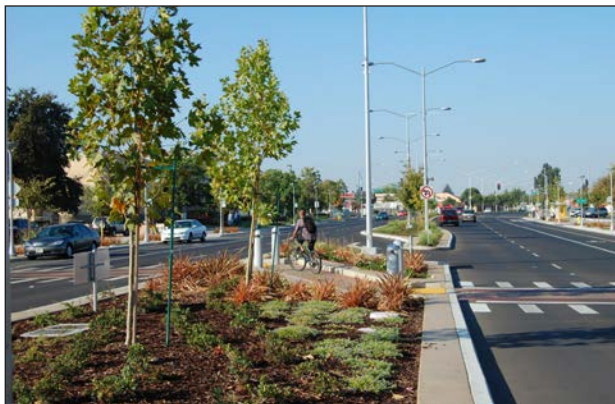
Median refuge island in West Sacramento.
