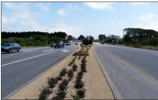
Median on Highway 1 in Half Moon Bay is designed with low maintenance, drought-tolerant landscaping. High contrast materials increase visibility to motorists.
