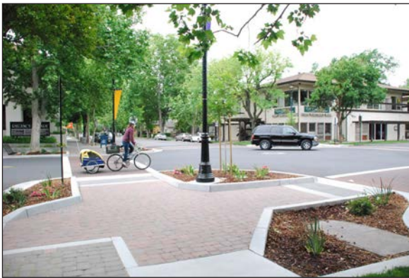
Curb extension in Davis, Ca.
