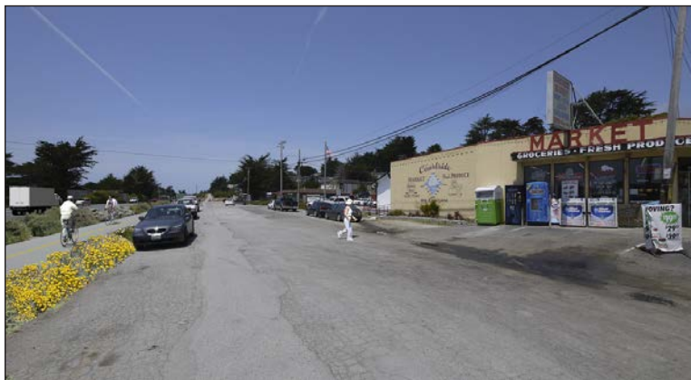
Carlos Street with the addition of the parallel trail with a landscaped buffer.
