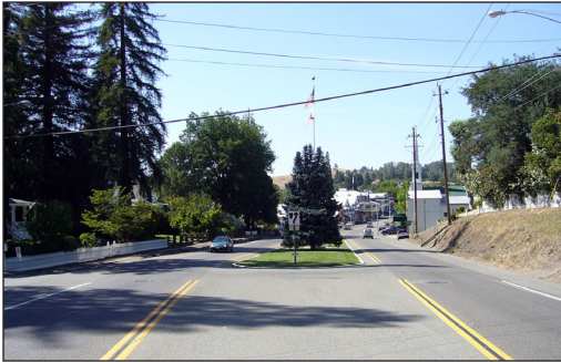
Median in Sutter Creek serves as a traffic calming entry feature into the town center.
