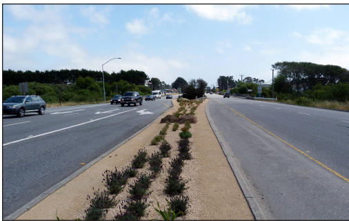
Median on Highway 1 in Half Moon Bay is designed with low maintenance, drought-tolerant landscaping. High contrast materials increase visibility to motorists.
