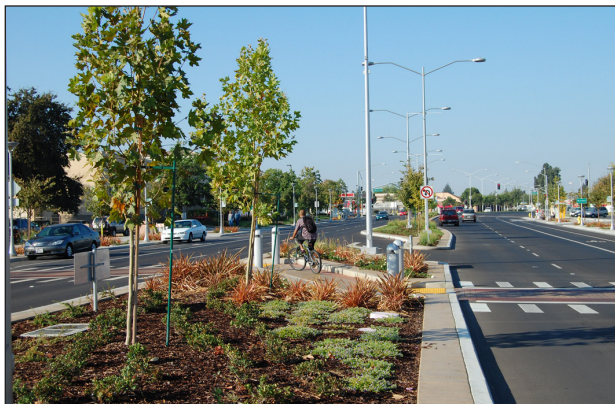
Median refuge island in West Sacramento.
