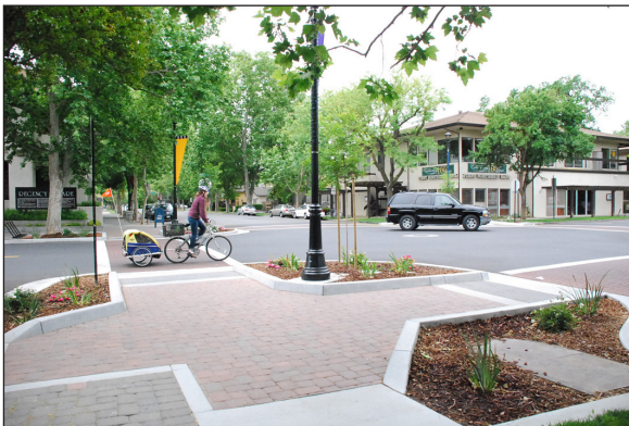
Curb extension in Davis, Ca.
