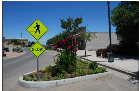
Landscaped curb extension and signage on Main Street contributes to traffic calming and beautification.
