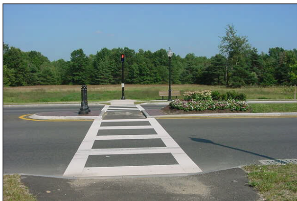
Pedestrian crossing island.
