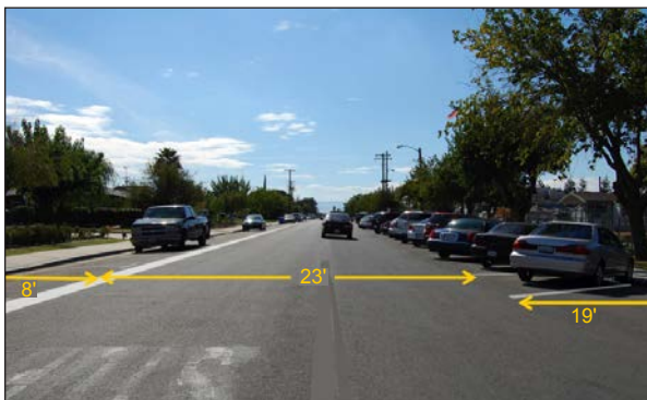
9th Street, with the center line removed, parking stalls lengthened and a solid stripe designating parallel parking. The narrowed travel way will encourage slow speeds.
