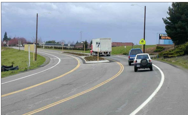
The photo above shows how a median crossing island can contribute to traffic calming by visually narrowing the roadway.
