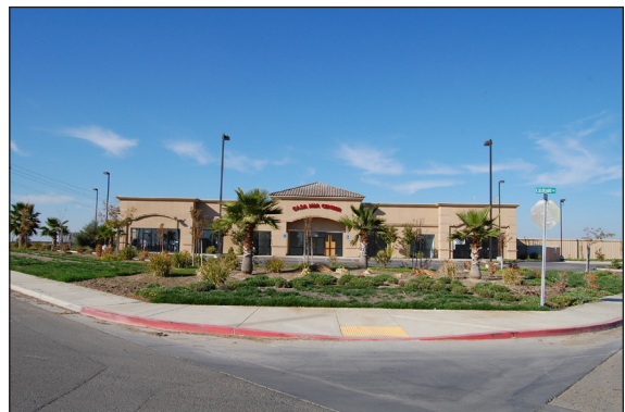
Recently constructed small retail building on Colorado Avenue remains vacant.
