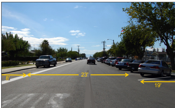
9th Street, with the center line removed, parking stalls lengthened and a solid stripe designating parallel parking. The narrowed travel way will encourage slow speeds.
