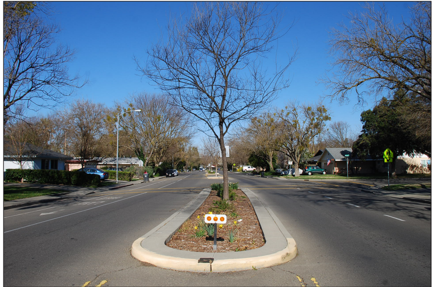
The photo shows an example of a median island with bike lanes and parallel parking on both sides of the street.
