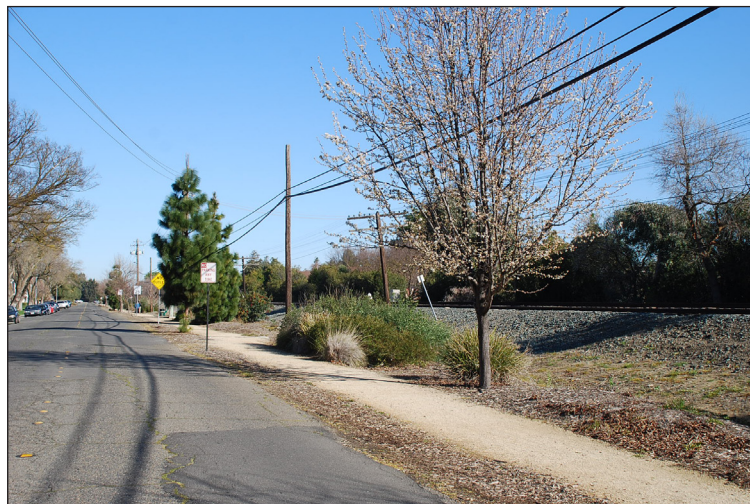
The photo above shows a potential short term option for Colorado Avenue that would include a trail with landscaping between the street and railroad tracks. The trail in the image above consists of decomposed granite.
