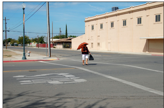
Long crossing and lack of shade at the intersection of Main Street and Nevada Avenue.
