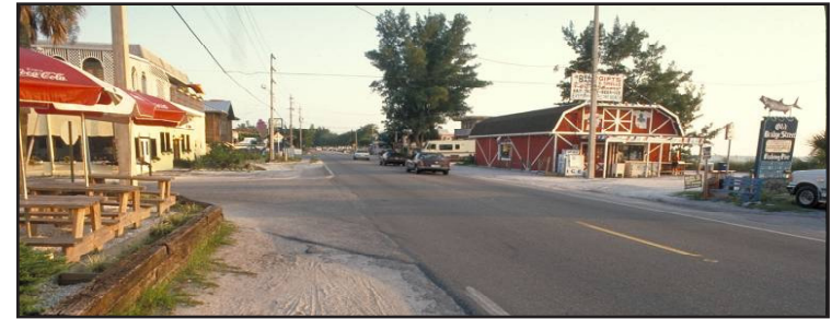
Bradenton Beach, Florida. This high-volume intersection was one of the town’s most dangerous for pedestrians, though immediately adjacent to its prime amenity.
