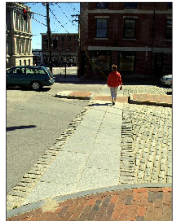
Tactile edges allow the vision-impaired to sense the edge of the “safe zone” for pedestrians and know they are crossing traffic.
