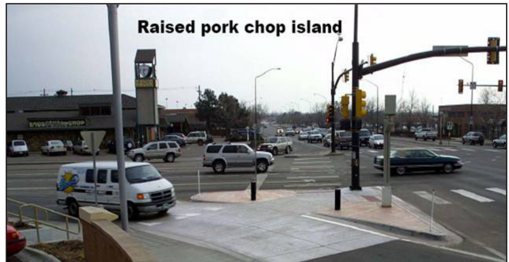
The photo to the right illustrates a low speed entry ramp accentuated by a raised crossing to assure low speeds.
