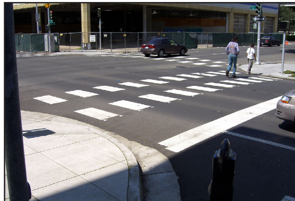
Crossings can feature high-visibility striping.
