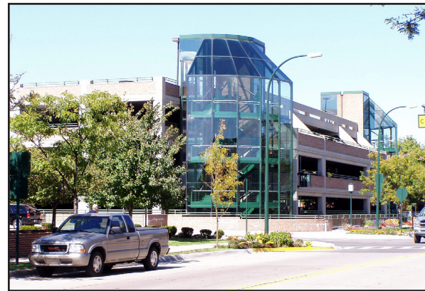
This garage has transparent stairwell walls for increased safety.
