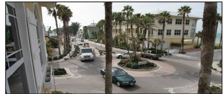
Installation of a roundabout calmed traffic speeds and facilitated pedestrian crossing. It also improved property values and catalyzed redevelopment.
