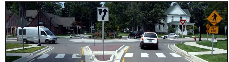
Myth breaker. This Brighton, Michigan roundabout disproved the myth that roundabouts with dominant primary street volumes will not let side street traffic enter during peak periods. It handles 20,000 vehicles per day and vehicles on the secondary street find numerous gaps when cars enter or exit the roundabout, a pedestrian crosses or a cars slow to park.
