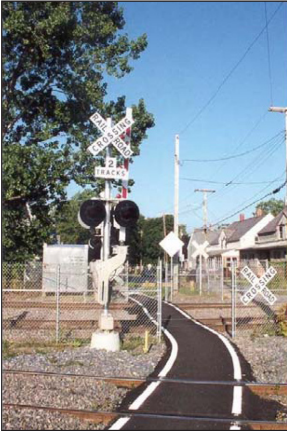
Examples of an At-Grade Rail Crossing. Source: Flickr user Eddie from Chicago under a Creative Commons License.
