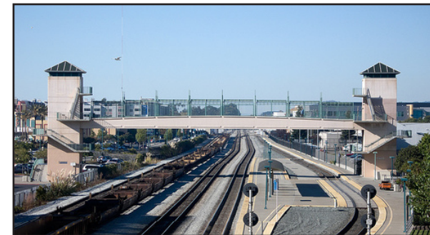
Example of Above-Grade Rail Crossing. Source: Flickr user Spacedust2019 under a Creative Commons License
