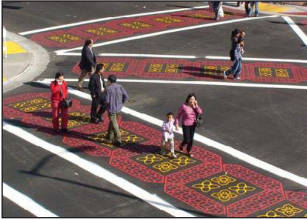
Example of Pigmented Asphalt at Pedestrian “Scramble” Crosswalk. Source: Integrated Paving Concepts.
