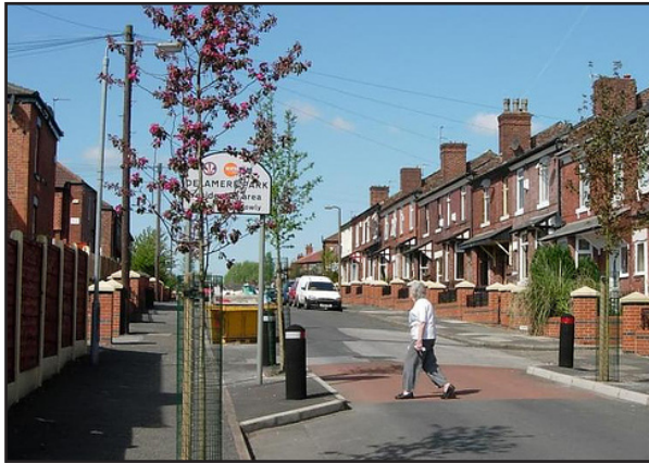
Example of Mid-block Pedestrian Bulb-out and Crosswalk. Source: Flickr user Greenstreeter under a Creative Common License.
