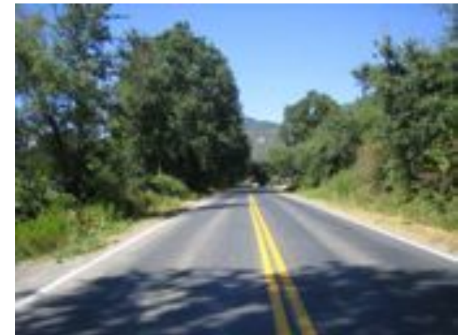
Mina Road (looking north).
