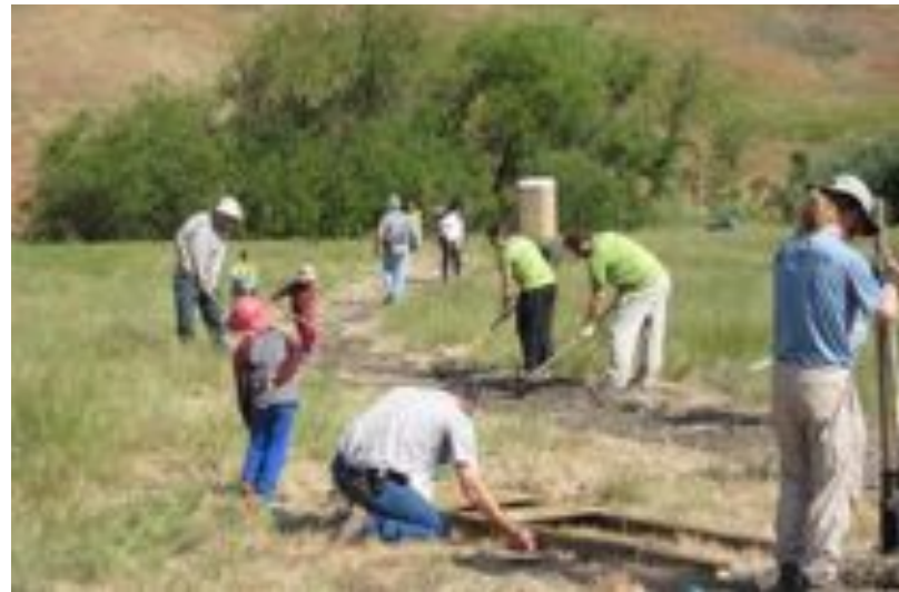
Community trail construction project.
