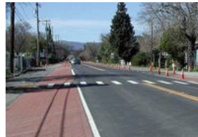
Examples of highly visible painted crosswalks and special paving used for shoulders. These treatments slow vehicles down and make streets more pedestrian friendly.
