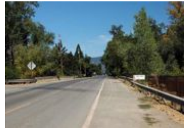
Hwy 162 Bridge over Towne Creek has wide shoulders for pedestrians and cyclists.
