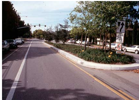
Raised medians, similar to the one above, are proposed along the SR108 corridor. Plantings are carefully selected to ensure they do not limit driver visibility.
