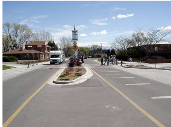
Bulb-outs, a short raised median, and a raised speed table provide a safe, convenient crossing for pedestrians.
