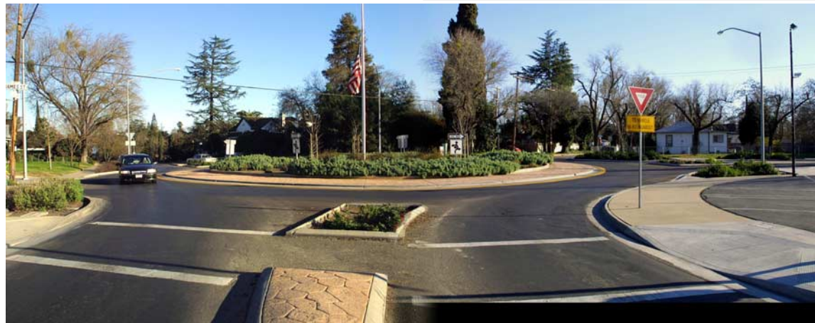
This roundabout at G Street and La Loma in Modesto handles 20,000 cars each day. Pedestrians wait for a gap in traffic or for a driver to stop, then cross to the refuge area.
