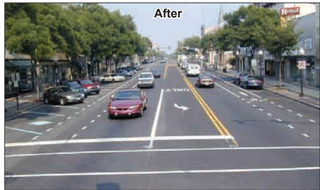
Two travel lanes are removed and replaced with bicycle lanes and angled parking on one side, increasing the number of on-street parking spaces.
