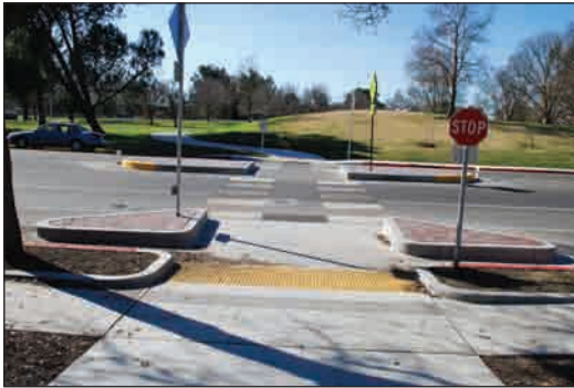
This trail crossing includes low maintenance curb extensions and crossing island.
