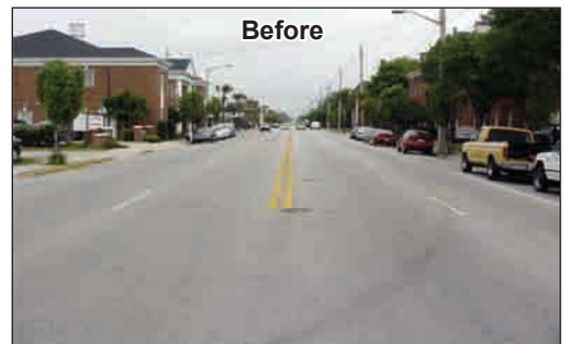
A four-lane road before a road diet.
