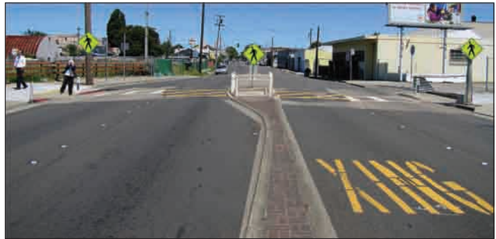
The photo simulation shows the impact of the addition of a small median with a wider refuge area and crossing signage. The crossing island includes lean bars for bicyclists.
