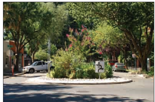
Top to Bottom: Curb extension with diagonal parking on Macdonald Avenue. Extension with curb cut for stormwater drainage and infiltration. Mini-circles in a series slow traffic on a Seattle street. A landscaped traffic circle in Sacramento.
