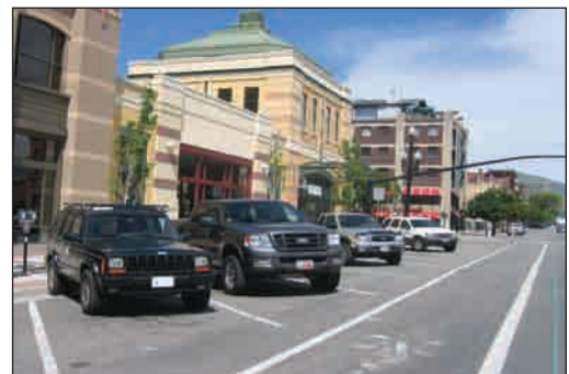
Back-in angled parking in Salt Lake City, with vehicles facing the bike lane.
