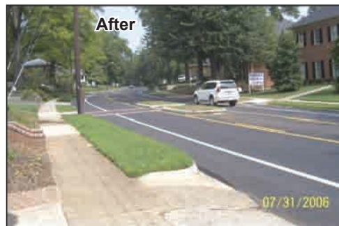
A road diet creates space for a crossing island, where pedestrians can pause before crossing the next lane of traffic. Crossing islands encourage motorists to yield to pedestrians.
