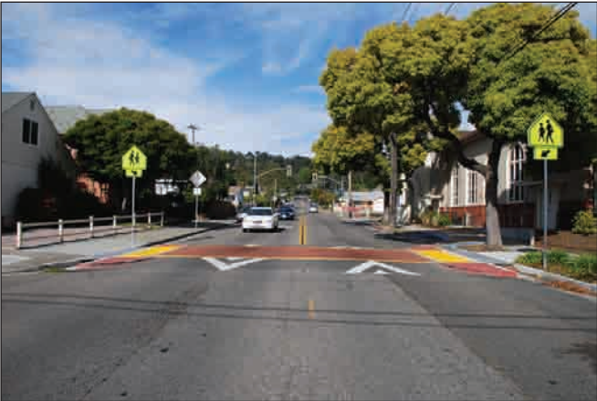
Example of a raised crosswalk at a school in El Cerrito. The raised crosswalk heightens the prominence of the crossing and provides a speed table that slows motorists. A similar type of treatment could be used near schools and other locations in Richmond with high crossing demand.
