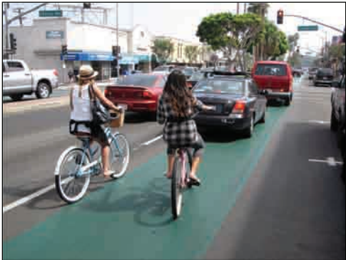
6-foot painted green sharrow centered in the right travel lane on 2nd Street in Long Beach, Ca.
