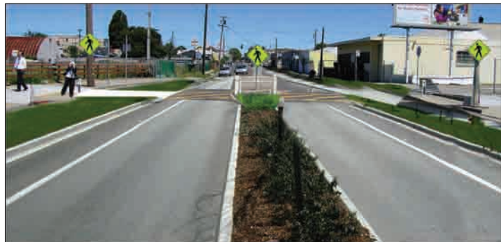
The photo simulation shows the crossing with the replacement of a travel lane in each direction with wider sidewalks buffered by green strips, which greatly improves the visibility to motorists of people on foot or bicycle preparing to cross. The narrowed travel way will encourage driver caution and likeliness to yield. The road diet also enables a median wide enough to accommodate landscaping.
