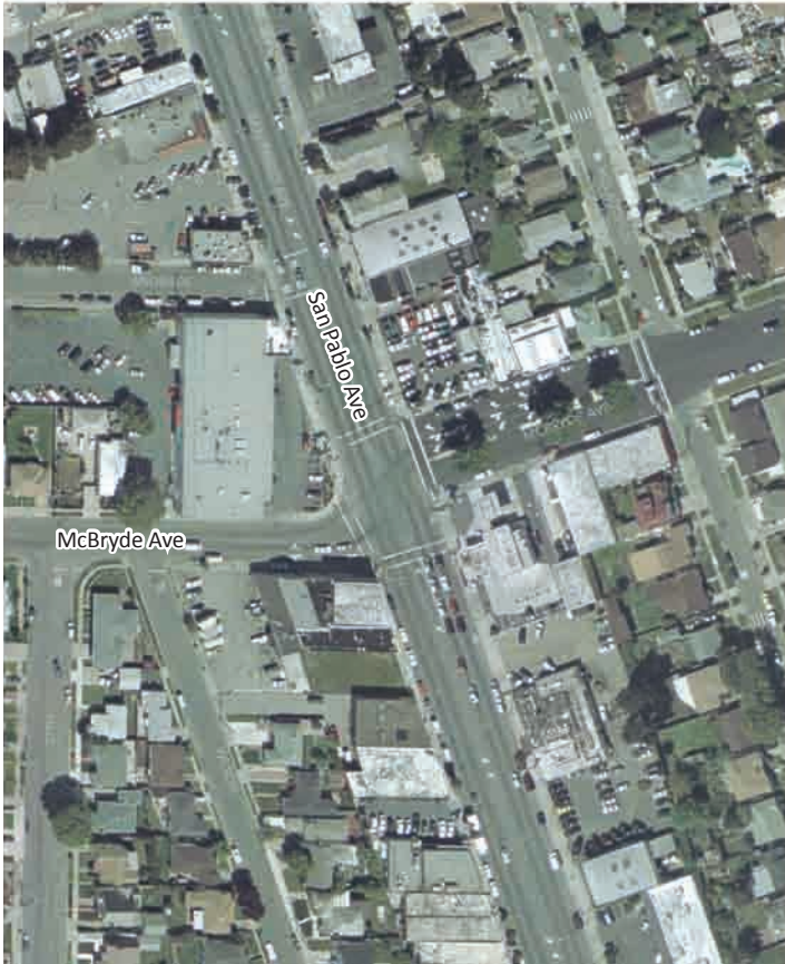
San Pablo Avenue at the intersection with McBryde Avenue.
