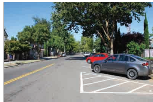
Back-in angled parking on a mixed commercial and residential street in Sacramento.
