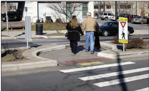
Angled refuge area directs attention to oncoming traffic.
