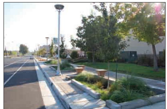
Planters with inlets to receive runoff in West Sacramento.
