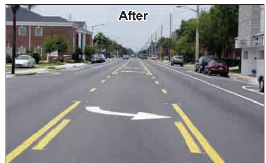
The same road is re-stripped with two travel lanes, a center turn lane, and bicycle lanes.
