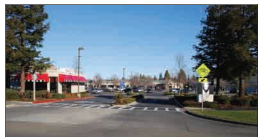
Larger driveway openings can be divided into right turn in and right turn out sections to reduce conflicts between turning vehicles and between vehicles and pedestrians. Crossing treatments can be added to send a clear message to drivers that they are crossing a sidewalk.
