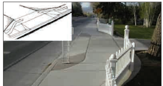
Where sidewalks are narrower it is sometimes possible to wrap the sidewalk around the driveway apron.
