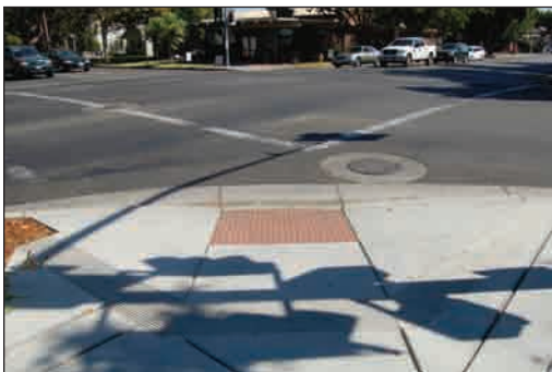
Single diagonal curb ramp.
