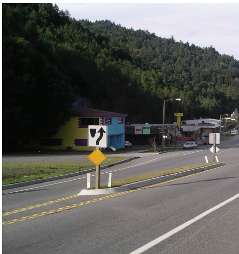
This photo illustrates a raised refuge median proposed for the Lunblade Street intersection.
