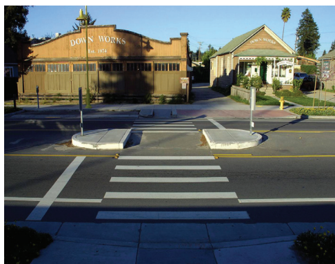
Example of raised medians at crosswalk locations that allow a refuge for pedestrians crossing a roadway with two-way traffic.
