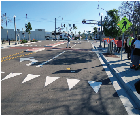
Shark's teeth indicate the point at which motorists are supposed to yield (or stop) for pedestrians.
