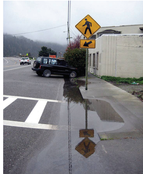
The crosswalk in front of the Orick theatre is submerged through the rainy season.
