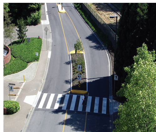
Warning sign along with a high visibility crosswalk and a raised median island inform the motorist of pedestrians.
