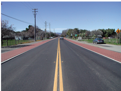
Colorized shoulders, like the one shown above on State Route 16 through the town of Capay, slow motorists down.
