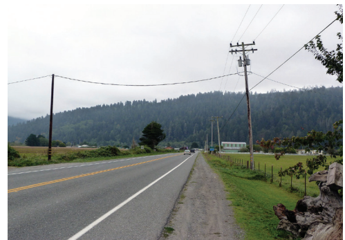
Approach from the south
