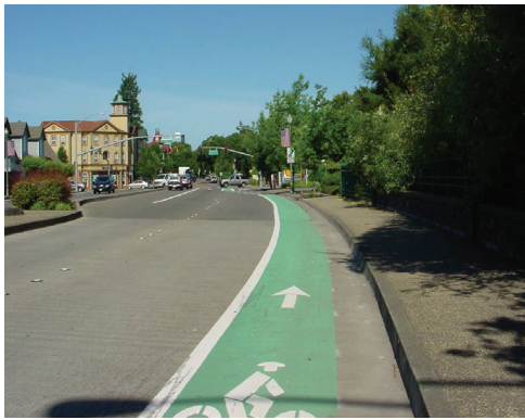
Bicycle lanes in the center of town could be highlighted by coloring them green as shown in this photo.
