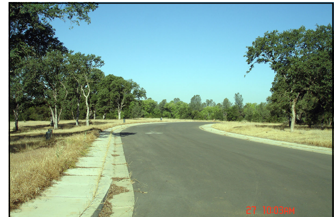
Roads and utilities have been installed to serve 42 additional housing units.
