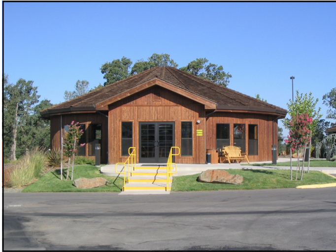
Traditional "roundhouse" architecture is reflected in the KOA Office building.
