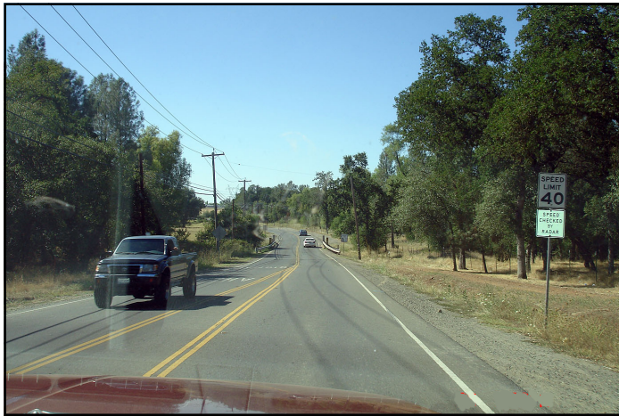
Narrow shoulders and lack of sidewalks makes walking to school difficult and unsafe.
