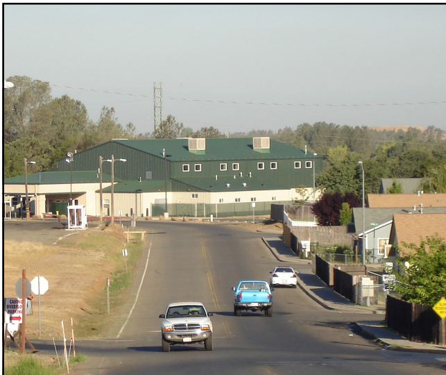
The straight alignment and overly wide road on Alverda Drive supports speeds in excess of the 25 mph posted limit.
