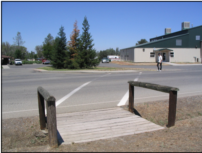
This crosswalk is located on a blind curve and is faded and difficult to see.
