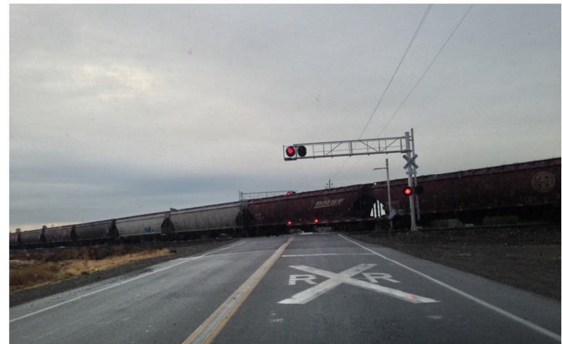
Freight trains frequently stop across Plainsburg Road and Childs Avenue, preventing pedestrian, bicycle, and auto access
