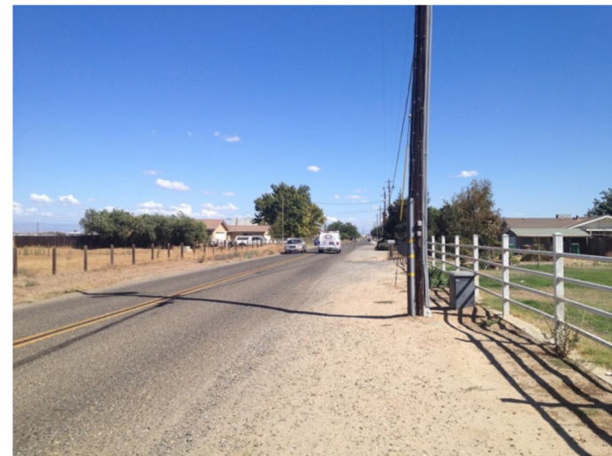
Sidewalks are missing on some of Franklin-Beachwood's primary roadways, including Dan Ward Road
