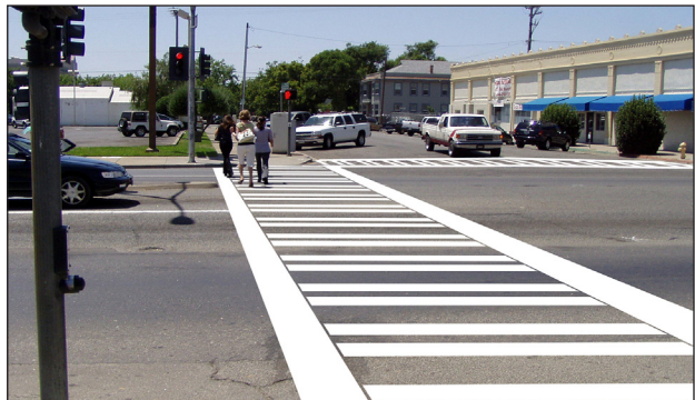
Above, left: Pedestrian view of existing E Street crossing. All signalized intersections should have high-contrast “ladder-style” crosswalks, like those shown in the photo simulation to the right.
