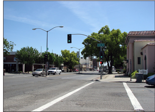
Crosswalk marking is inconsistent, as shown in the photo above. Crossing E Street here is legal, though the crosswalk is not marked, while the shorter 4 th Street has a marked crosswalk.
