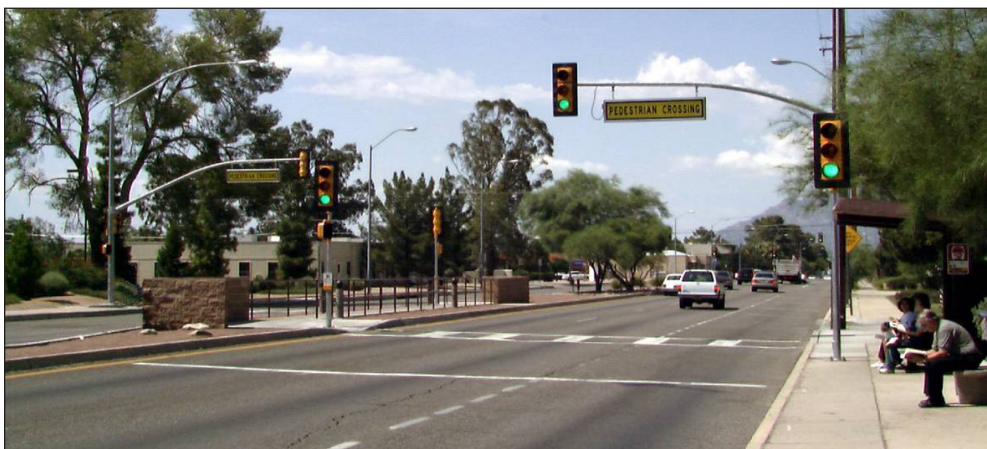
The photo above shows a two-stage pedestrian crossing. After the first stage, crossing to the center island, pedestrians must walk to face traffic before completing the second stage. A signal, as shown above, is not required for two-stage pedestrian crossings.
