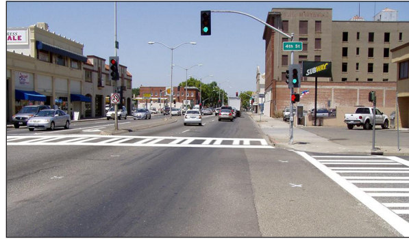
The motorist's view of the same intersection and simulated crosswalk markings. High-contrast markings alert drivers to watch out for pedestrians. Ladder-style markings are spaced so that vehicle tires travel between crossbars, instead of over them. This reduces wear and maintenance of crosswalk markings.
