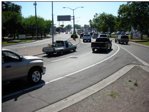
10 th Street at the curve north of E Street. Note the vehicle in the right turn lane. The right “trap lane” drops before the bridge. During field observations, few vehicles turned right from the lane. Most merged into through traffic lanes to cross the bridge. This movement is sometimes erratic. Conflicts are created as drivers attempt to pass as many cars on the right as they can before entering the traffic stream.
