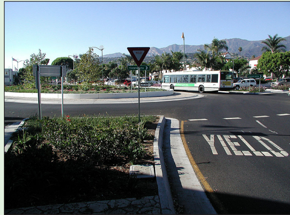
Roundabout size is dependent upon the volume and type of traffic that will pass through the intersection. Roundabouts can be designed to accommodate the largest trucks.
