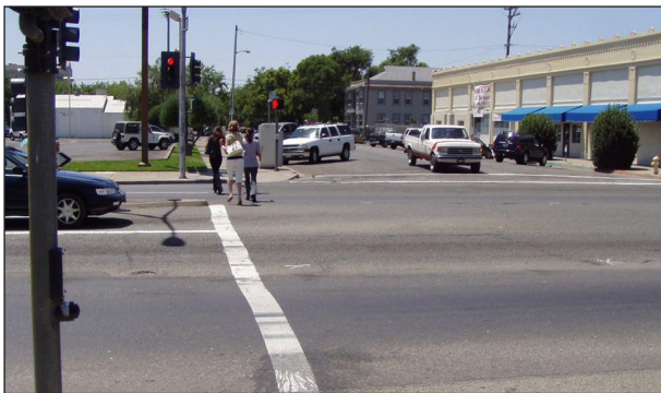
Above, left: Pedestrian view of existing E Street crossing. All signalized intersections should have high-contrast “ladder-style” crosswalks, like those shown in the photo simulation to the right.
