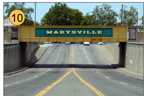
The railroad bridge on Highway 20 just east of Ellis Lake is an ideal gateway sign location.
