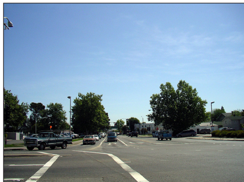
E and 9th Street is a busy, large intersection. Note the dogleg crosswalk. Also notice how far pedestrians have to cross.
