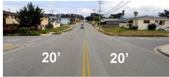
Reindollar Avenue – existing condition
