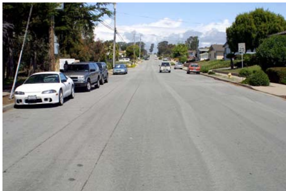
DeForest Road – existing conditions
