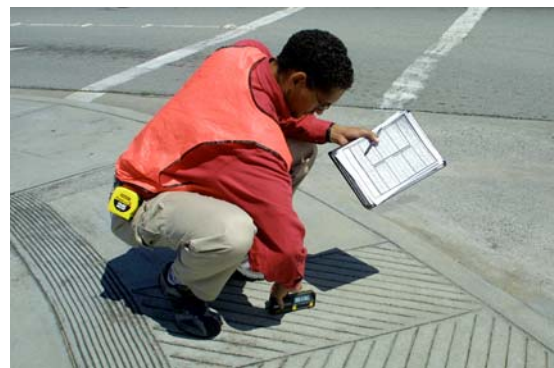
Several curb ramps had improper slopes and landings
