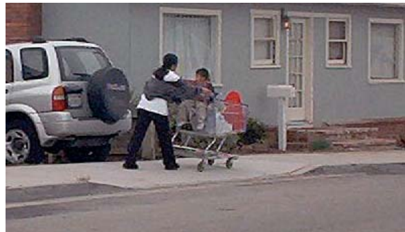
Improper driveway without planter strip – even mothers pushing strollers are negatively affected by the excessive cross-slope.
