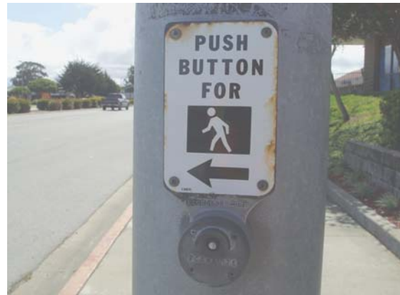
This pushbutton is too small – it should be 2” to be more easily used by all pedestrians
