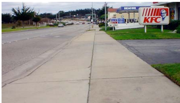
Proper driveway with “flat” area for sidewalk
