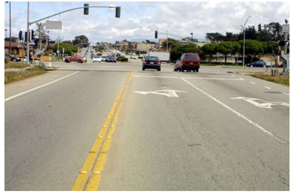
Existing Bike lanes on Reservation Road
