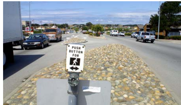
Signals should be timed so that pedestrians do not need to push a button in the median
