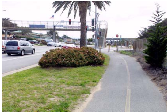
Trail adjacent to Del Monte Blvd.
