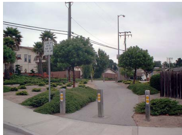
Pedestrian and bicycle connector at Barrett Lane in Marina
