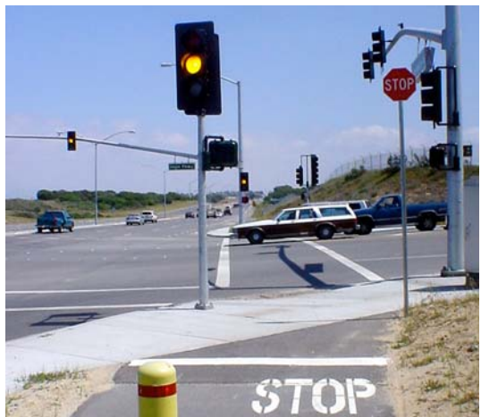
This stop sign should be removed
