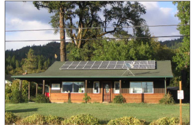
Figure 8-10 With abundant solar exposure, Laytonville could strive for energy-independence.
