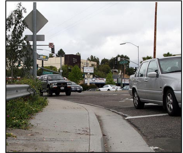
Westbound I-8 onramp with dangerous crosswalk.
