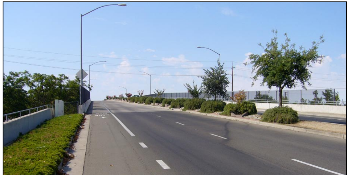
...because no raised sidewalk is provided on east side to preserve width for 4 vehicle lane option in future.
