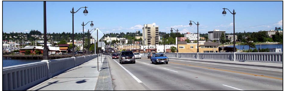
The 4th Avenue Bridge is still designed to carry significant traffic volumes.
