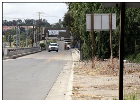
...and southbound bridges redesigned...
