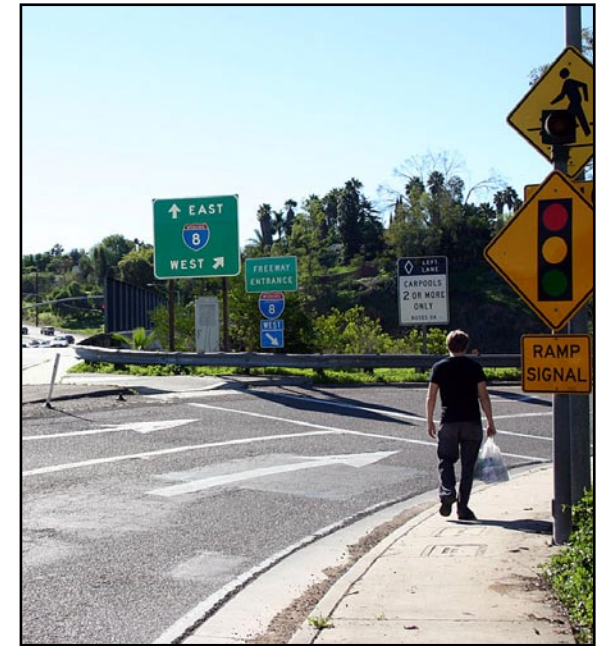
Pedestrians are obscured by the curve and poles.
