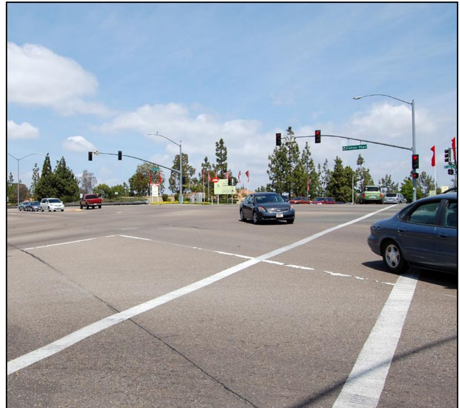
...encounter fast traffic, poor sight lines, and very long crossing distances.
