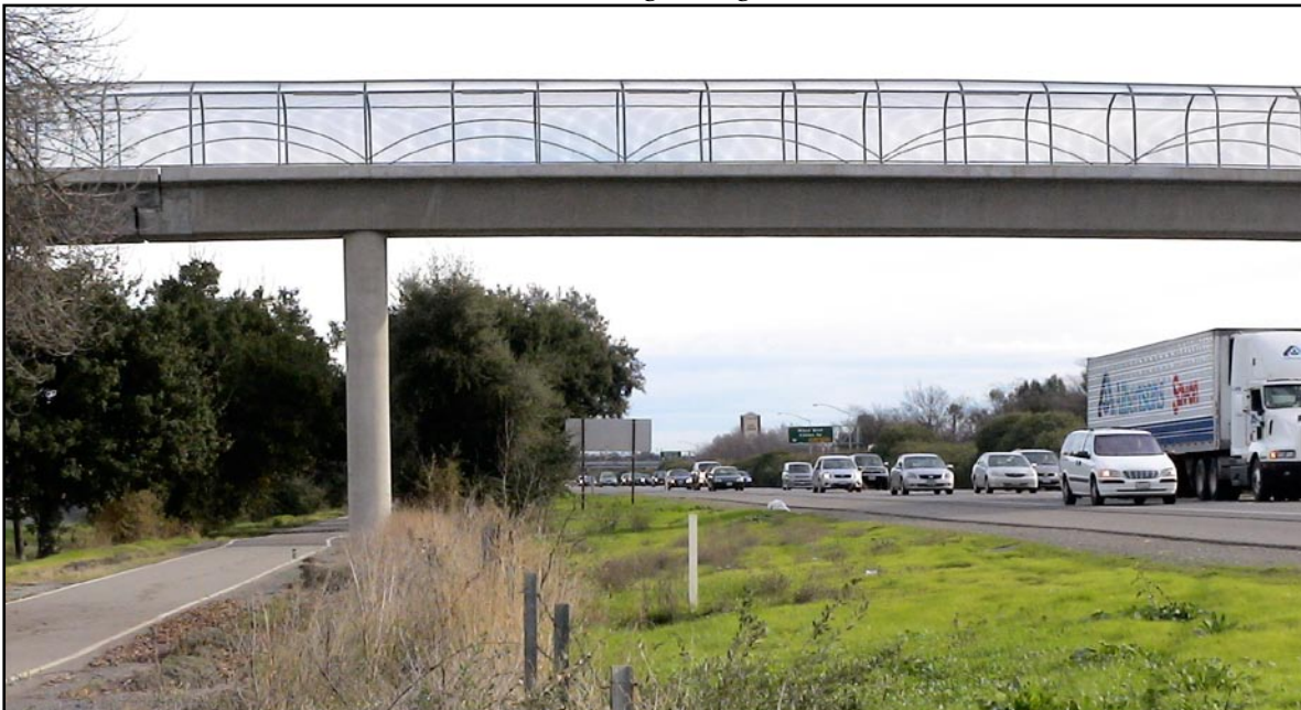
Dave Pelz Overcrossing, looking east, with bicycle path installed on old U.S. Route 40 pavement.
