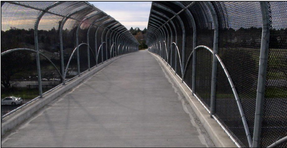
Dave Pelz Overcrossing, looking north (above).
