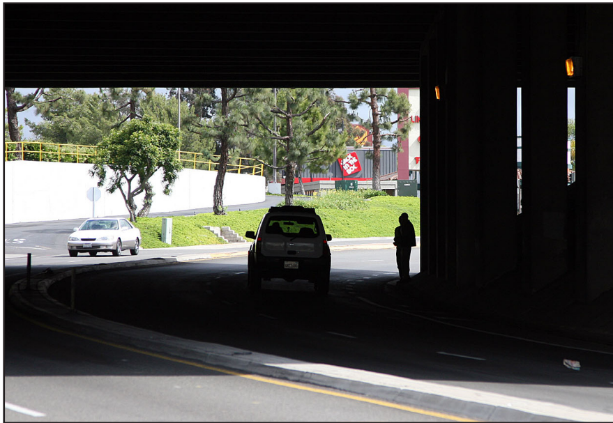
Narrow bike lanes on the inside of the dark curve are especially dangerous.
