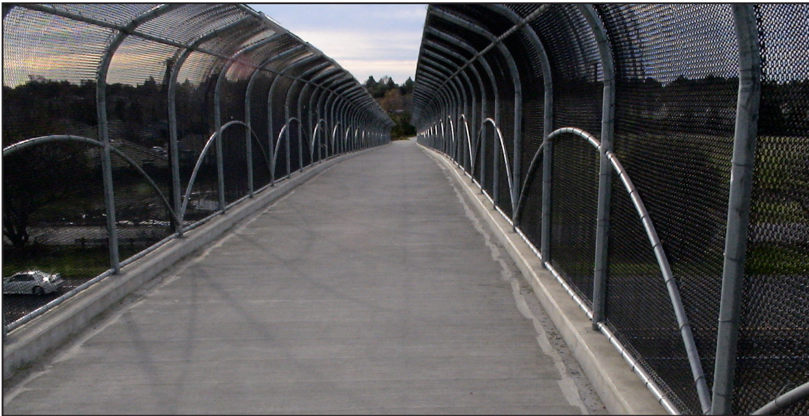
Dave Pelz Overcrossing, looking north (above).
