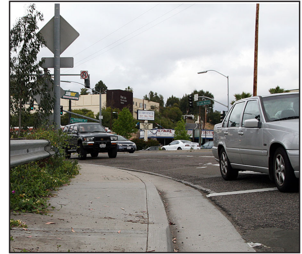
Westbound I-8 onramp with dangerous crosswalk.
