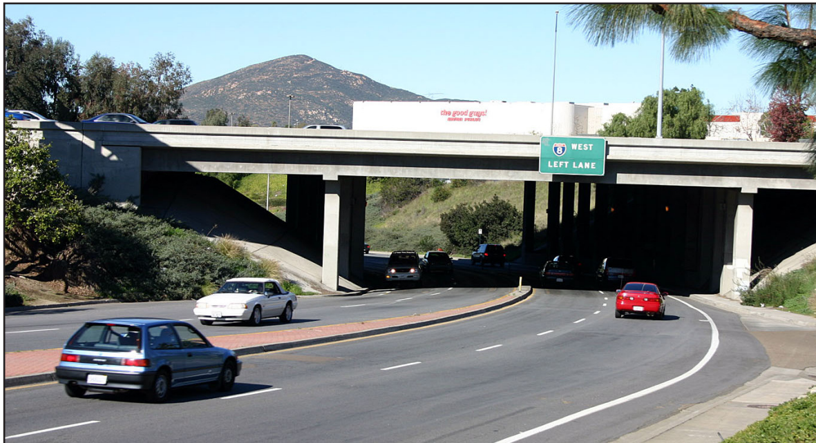
The Jackson Drive undercrossing with narrow and exposed bike lanes and only one sidewalk.
