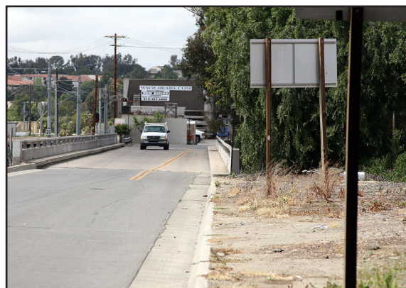
...and southbound bridges redesigned...
