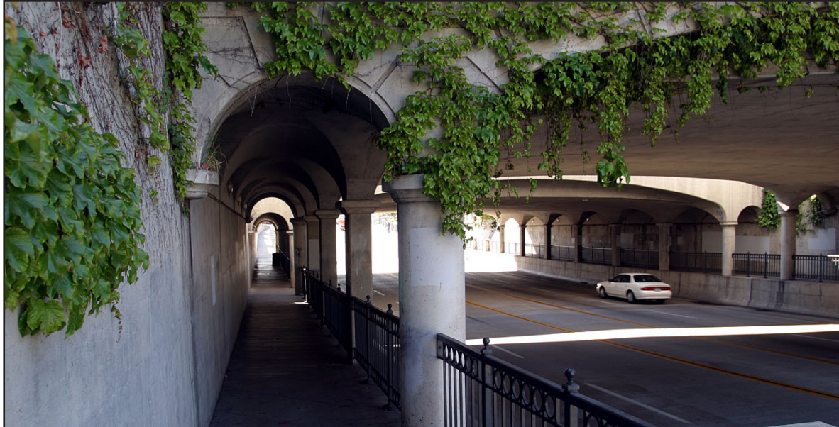
Raised sidewalk reduces drop and climb for pedestrians, and is much safer from automobile intrusion.
