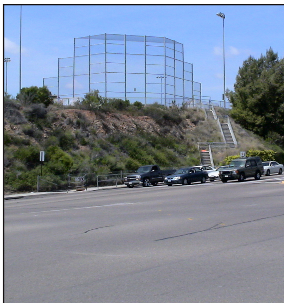
Previous short route used these stairs...
