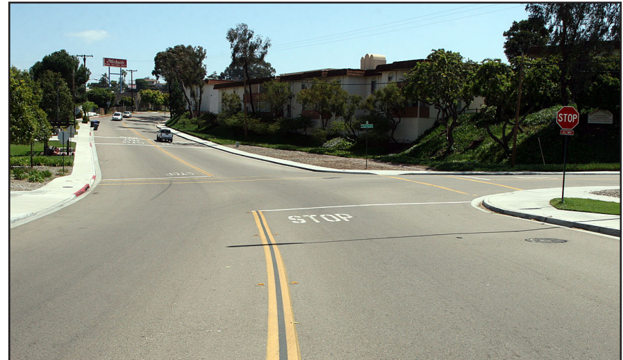
...this intersection needs curb extensions and highly visible crosswalks.
