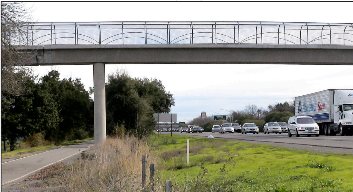
Dave Pelz Overcrossing, looking east, with bicycle path installed on old U.S. Route 40 pavement.
