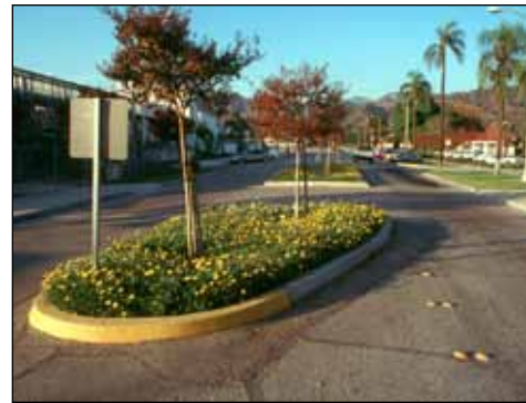
Crosswalk cut through a median provides a pedestrian refuge.
