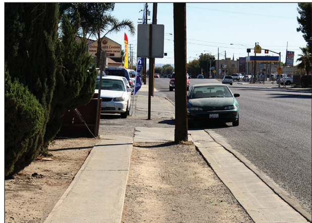
Some portions of sidewalks along Lassen Avenue are inconsistent or have obstacles in the pathway.
