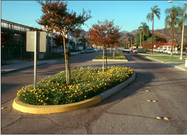
Crosswalk cut through a median provides a pedestrian refuge.
