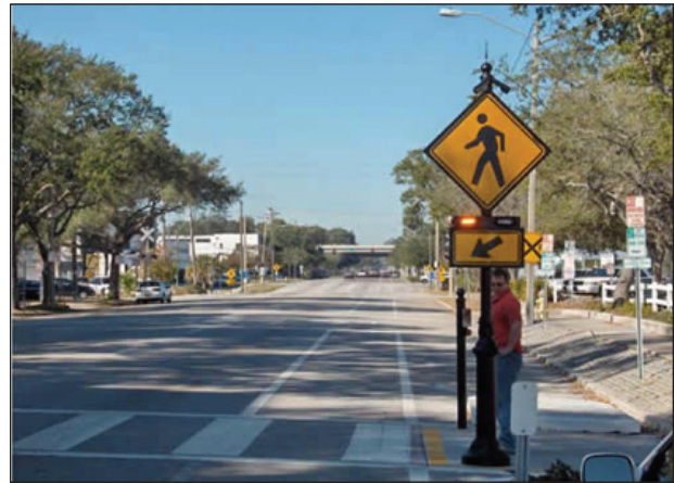
A rectangular rapid-flash beacon from the driver's point of view. Source: MUTCD, FHWA.
