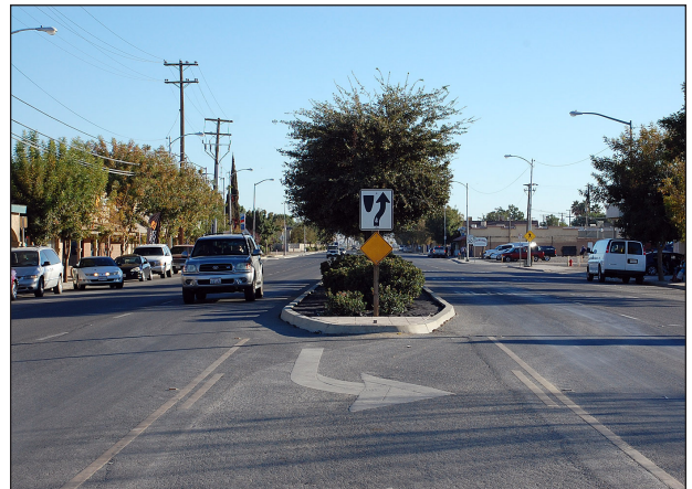
The City has added landscaped medians on the southern portion of Lassen Avenue.
