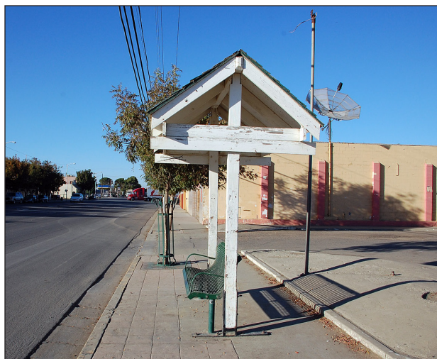
Nothing identifies this shelter near West America Bank as a transit stop.
