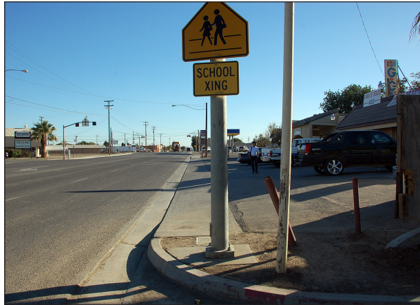
South of Corte Way on Lassen Avenue the sidewalk is missing an ADA compliant curb ramp and poles are in the pedestrian path.
