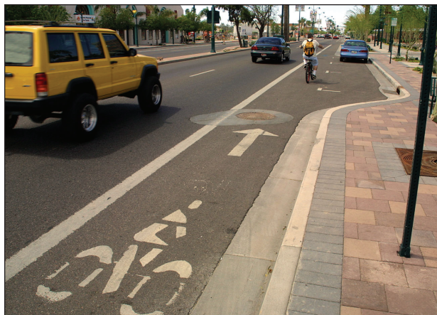
Bicycle lanes provide a buffer for cyclists between traffic and parked cars.
