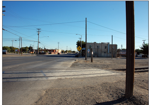
Sidewalks are missing in a few locations along Lassen Avenue such as this section north of Railroad Avenue on the west side of Lassen Avenue.
