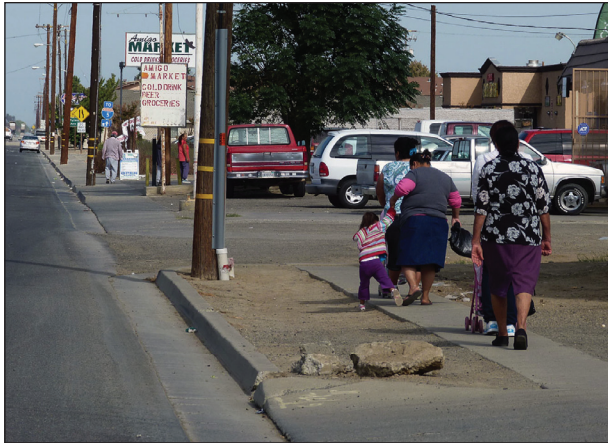
Mothers navigate substandard sidewalks on Lassen Avenue with strollers.
