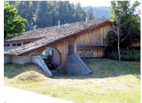
The Archives building reflects traditional building style and materials.
