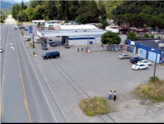
Uncontrolled access and egress can pose hazards to pedestrians as well as motorists.
