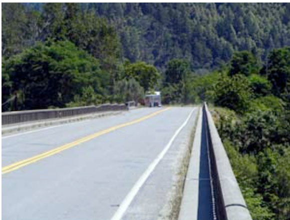
Trinity River Bridge—Before
