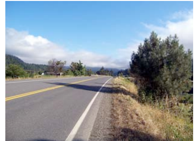
Highway 96 approaches the Trinity River Bridge northbound.
