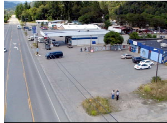
Uncontrolled access and egress can pose hazards to pedestrians as well as motorists.
