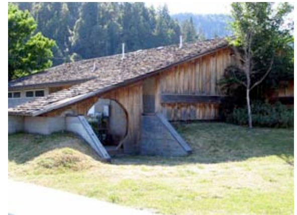
The Archives building reflects traditional building style and materials.
