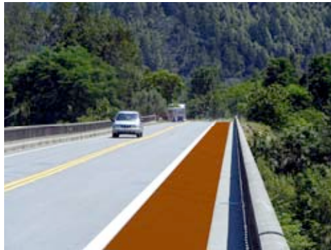
Trinity River Bridge—After
