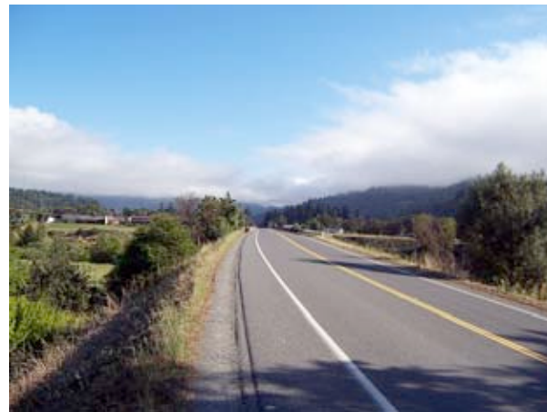
Northbound Highway 96 near the Trinity River Bridge and downtown Hoopa.
