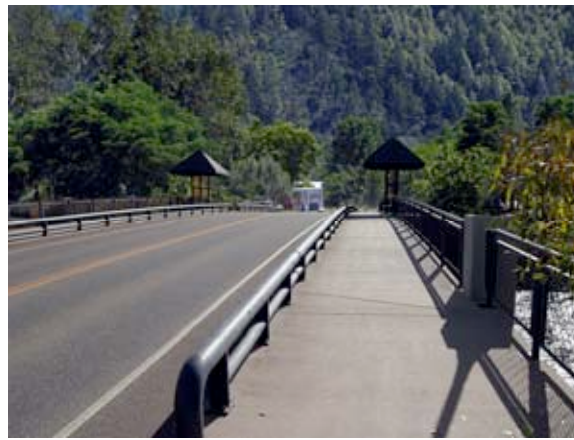
Trinity River Bridge—After
