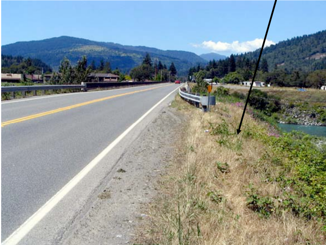
Highway 96 northbound approach to the Trinity River Bridge and Downtown Hoopa with possible locations of Gateway features.
