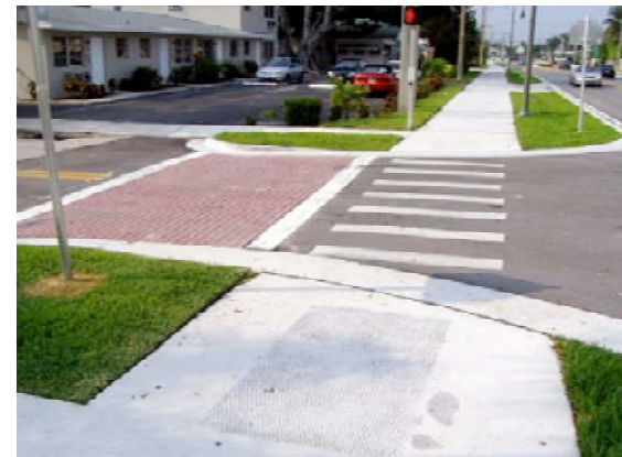
Well defined driveways help both pedestrians and vehicles in avoiding conflict.
