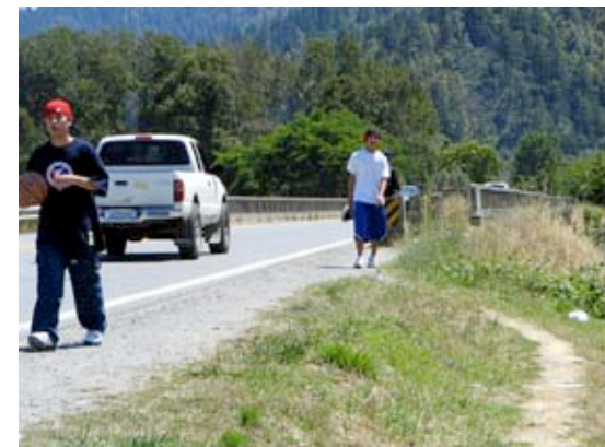
Crossing the bridge can be especially hazardous.
