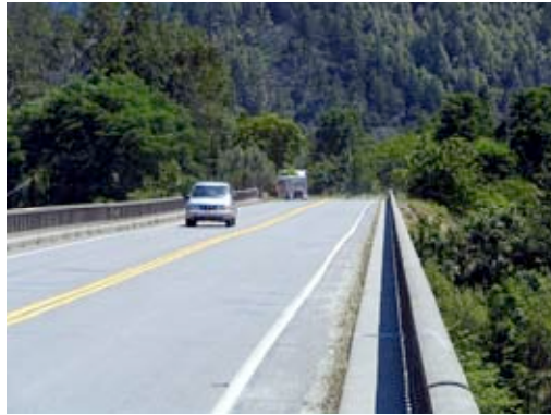
Trinity River Bridge—Before
