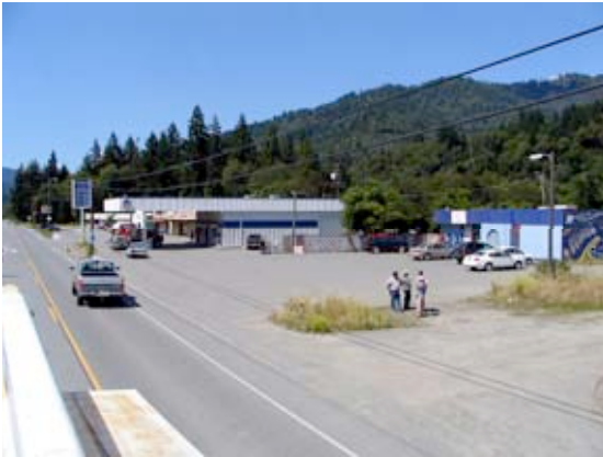
Access controls can direct traffic off and onto the highway.
