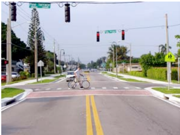
Pedestrian crosswalks should be highly visible to the oncoming motorist. Material and color changes help identify the pedestrian crosswalk along with appropriate signage.
