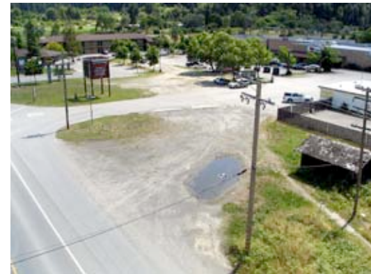
Access controls can eliminate short-cuts by vehicles.
