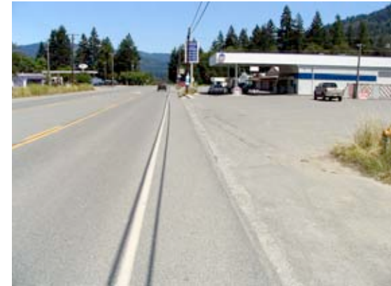
The lack of sidewalks poses hazards to pedestrians along the Highway.
