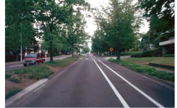
Bike lanes five feet wide can be provided between the parking area and travel lanes.
