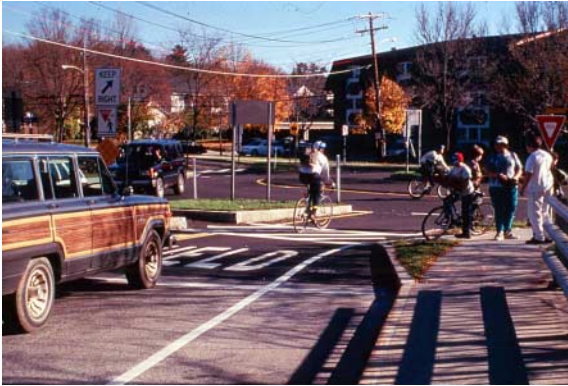
This Vermont roundabout is located adjacent to a school. Students benefit from the slower speeds and shorter crossings.
