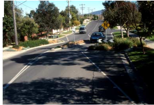
Angled slow points include extended curbs on the edges and a median between lanes. Drivers slow down to maneuver the curve this creates.
