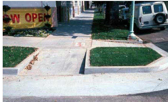
Two separate curb ramps are superior to one ramp angled at the corner. The style above provides excellent access for people in wheelchairs and also helps people with visual impairments identify the crossing area.
